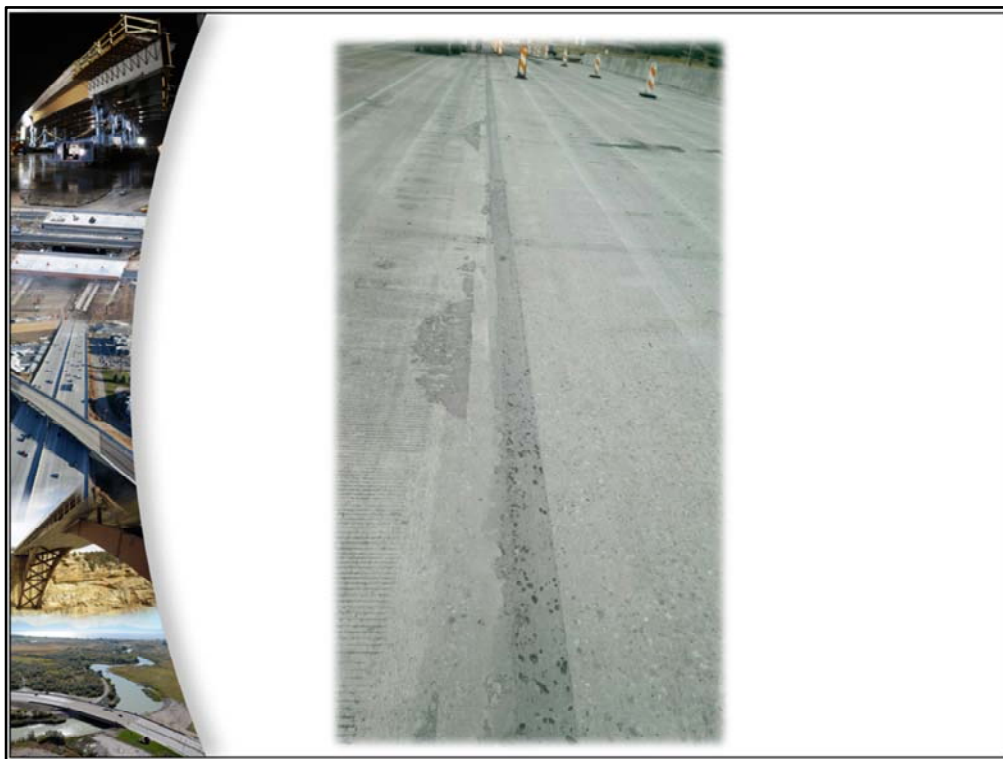
Longitudinal deck joint after being filled with UHPC.
