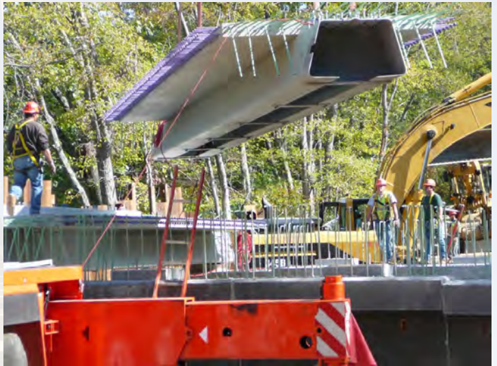
Installation of folded steel plate girder system at Uxbridge, Massachusetts
