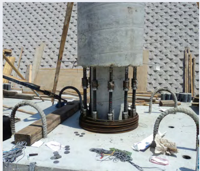
Headed bar couplers for precast column-footing connection
