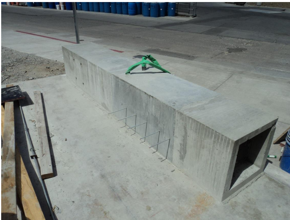
Precast concrete column
