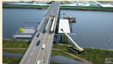
Permanent Span Erection
