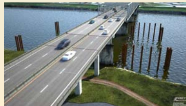
Open to Traffic – Temp Pile Remove
