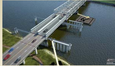
Temporary Piers – Permanent Span
