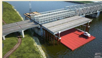
Skid in on beams
