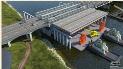
Float in on barges
