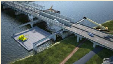
Temporary Piers – Temporary Span
