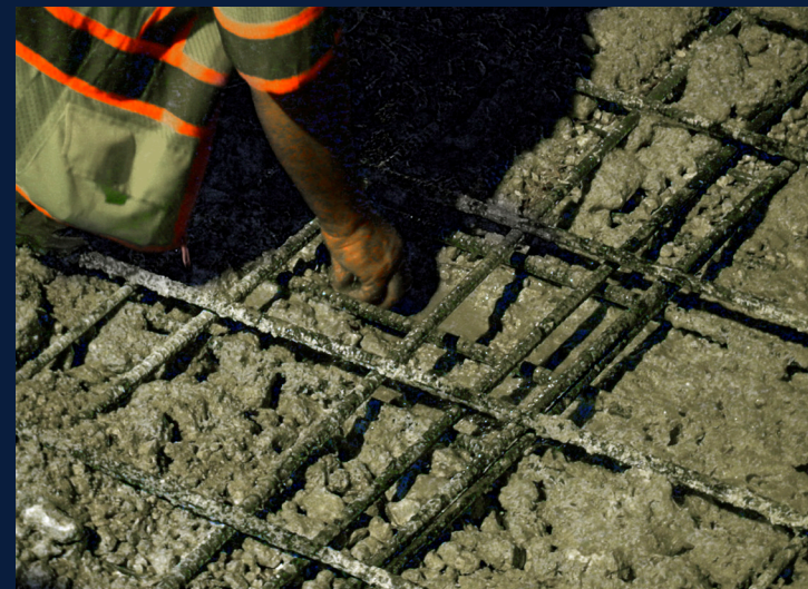
Example of hydro-demolition technique used to remove deck.
