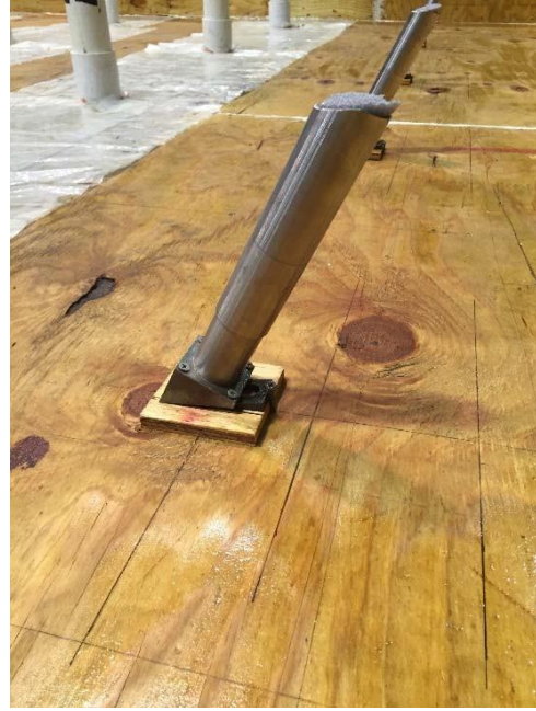
Figure 14 Inclined Bar Connection in Bridge Deck
