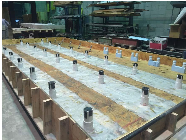
Figure 11 Concrete Beams with Deck Slab Formwork
