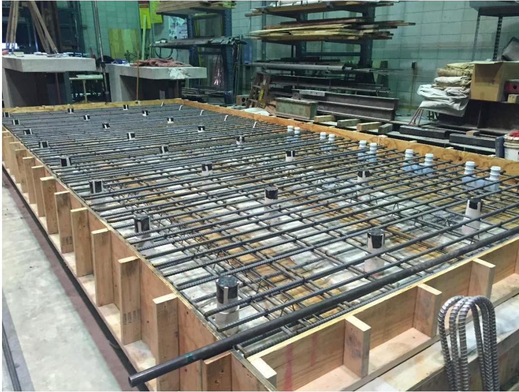
Figure 16 Bridge Deck Prior to Concrete Pour
