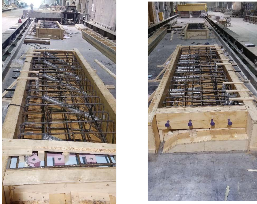
Figure 13 Precast Barrier Fabrication
