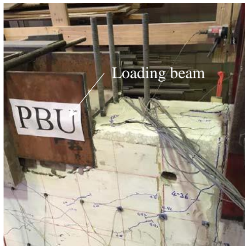
Figure 25 Cracking on barrier due to loading during Test 4
