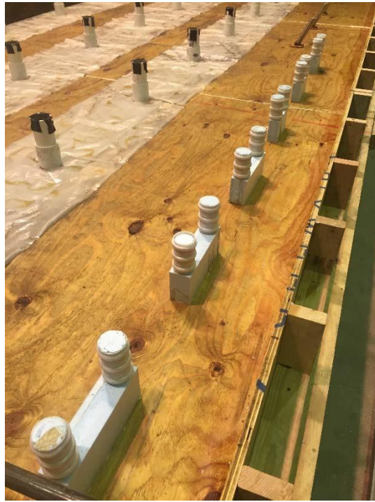
Figure 15 Pockets for U-bar Connection in Bridge Deck
