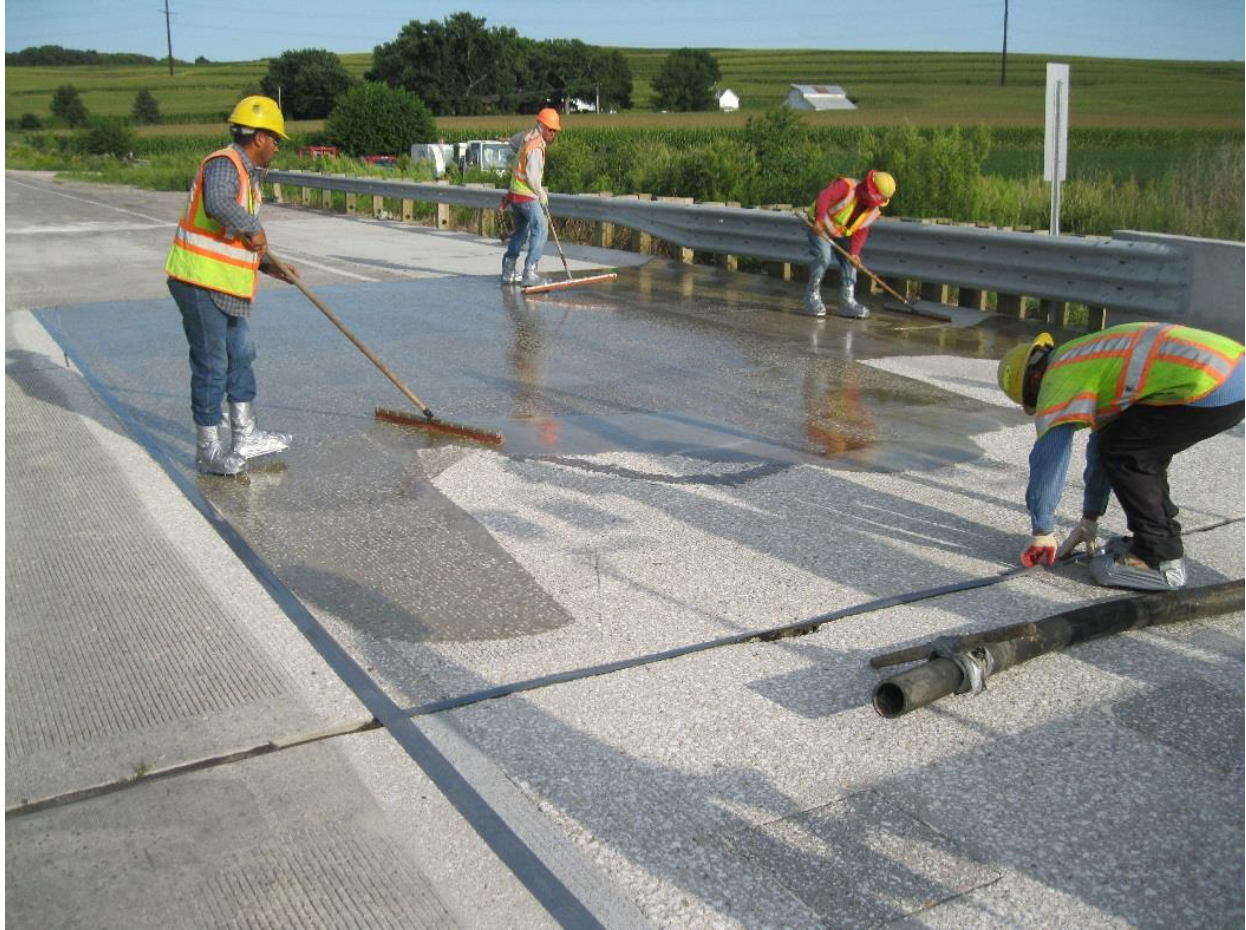
Figure 3. Polymer overlay application
