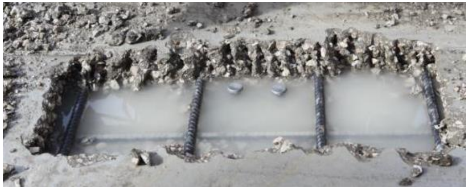
Phares et al. 2014, Bridge Engineering Center at Iowa State University
