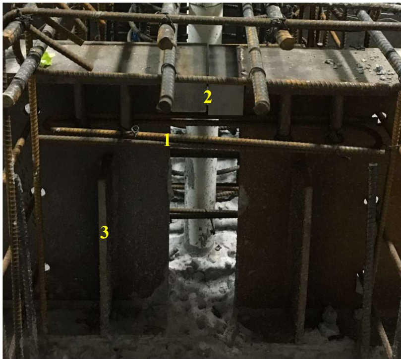
Figure 3-14 View of the connection detail as built.
