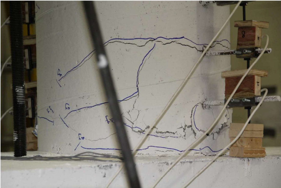
Figure 4-4 Crushing of concrete on the North side of the column at 1\Delta_y .
