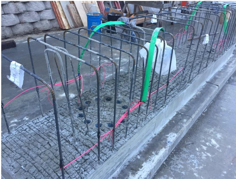
Fig. 46- Completed lower cap beam with corrugated ducts
