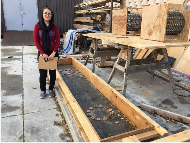
Fig. 40 – Formwork for the precast portion of cap beam
