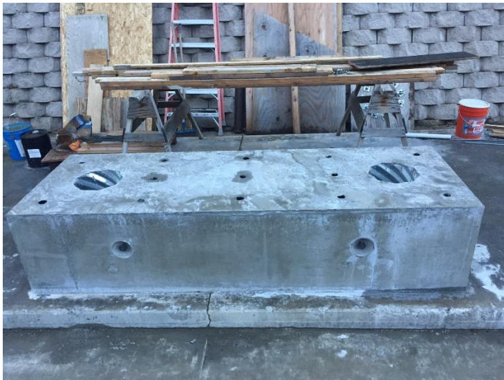
Fig. 44- Precast footing with sockets (pockets).
