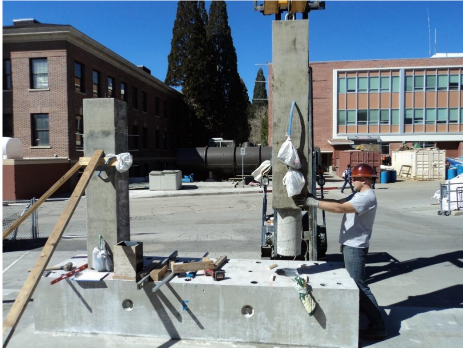
Figure 33. Inserting the second precast column into the footing
