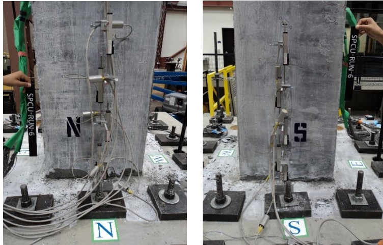
Figure 28. Damage state of the novel column after 200% design earthquake
