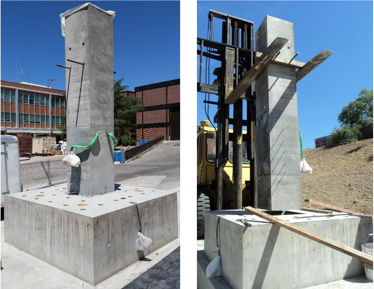
Figure 19. Insert precast column into the precast footing
