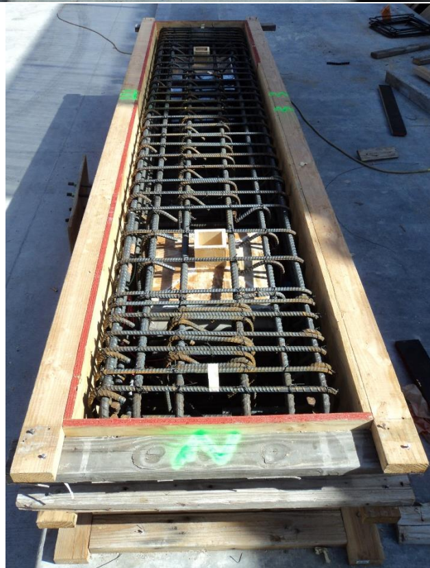
Figure 29. Cap beam construction and pocket for columns
