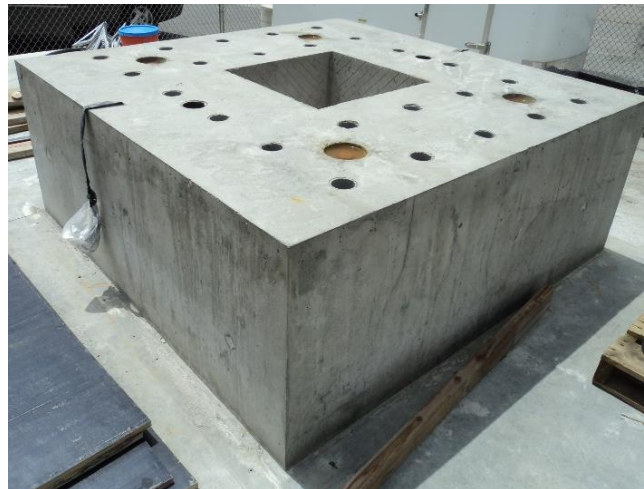
Figure 18. Precast footing with pocket area in the middle
