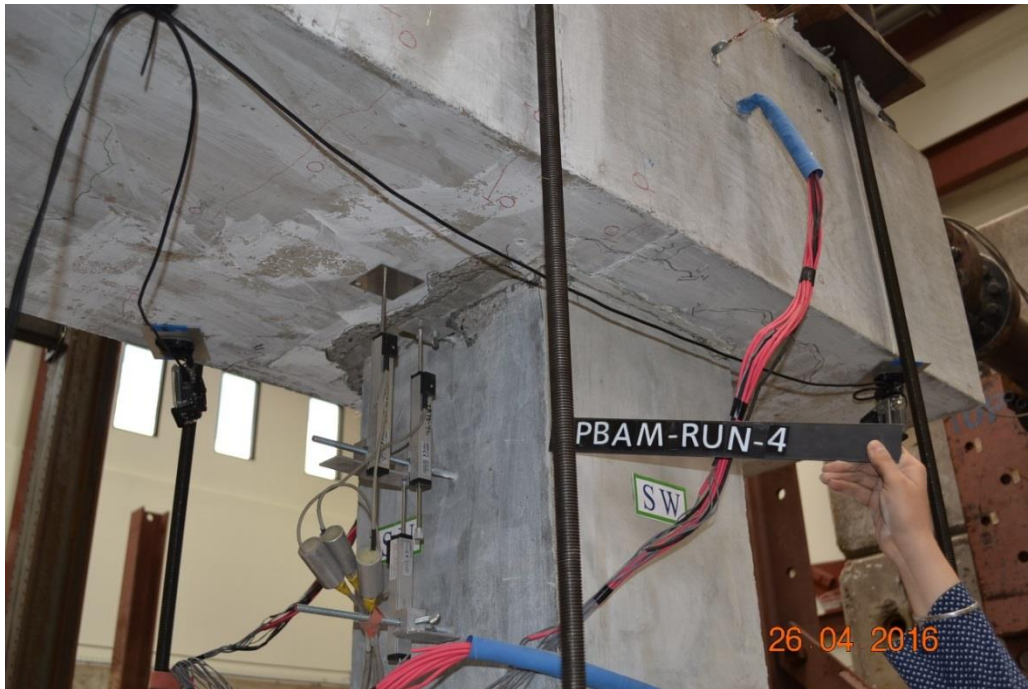
Figure 38. Damage state of UHPC plastic hinge and pocket connection under design motion
