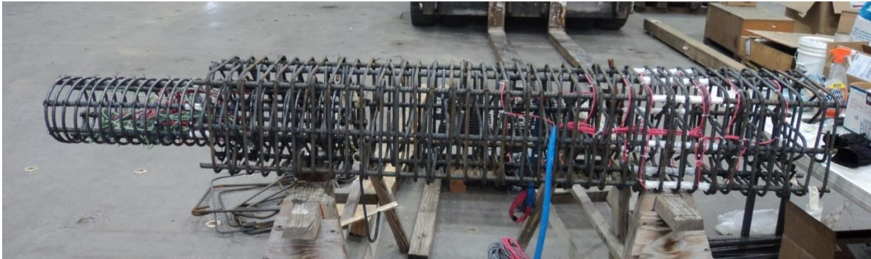
Figure 31. Column reinforcement cage
