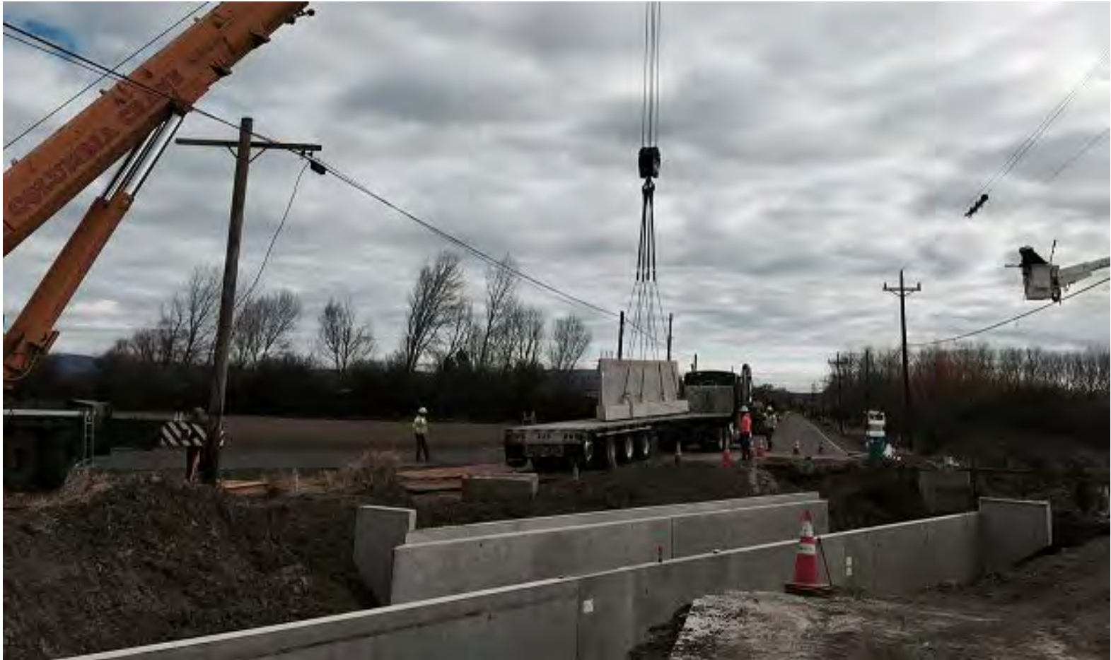
Abutment walls with footing being set
