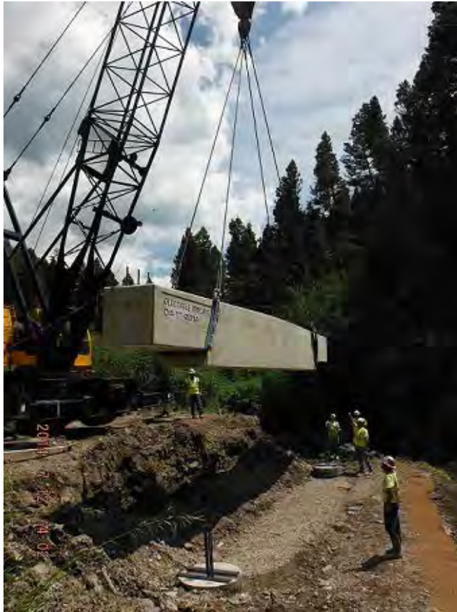
Pile cap being placed
