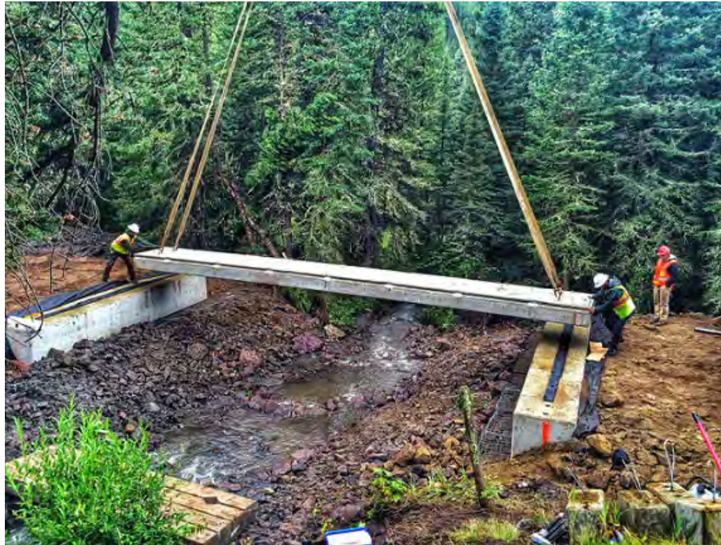
Slab set on grade beams
