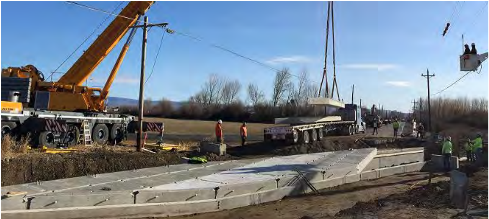
Deck being set
