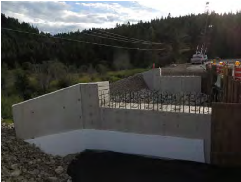
Willow pile cap
