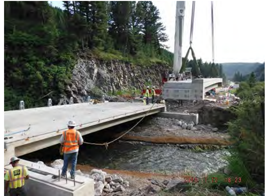
Deck being placed
