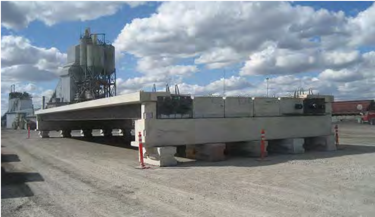
Trial fit in precast yard
