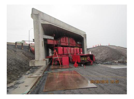
Climbing jacks hydraulic pump failure caused RSS wall to sustain load for 24 hrs
