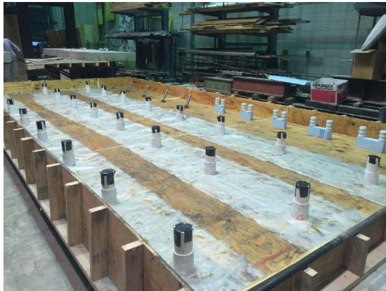
Figure 11 Concrete Beams with Deck Slab Formwork
