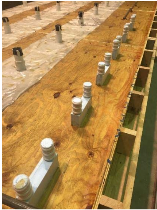
Figure 15 Pockets for U-bar Connection in Bridge Deck
