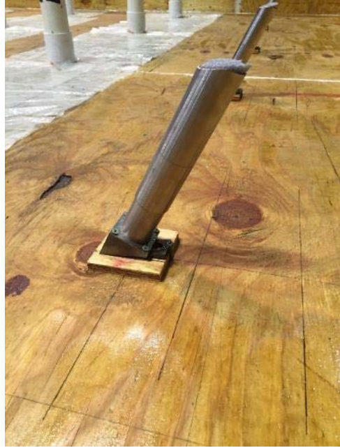
Figure 14 Inclined Bar Connection in Bridge Deck
