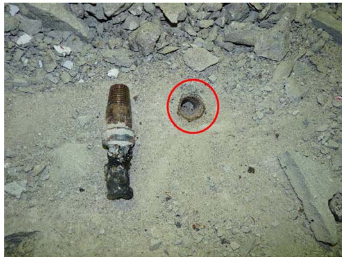
Figure 30 Removed Inclined Barrier Connection and Receiving Deck Piece
