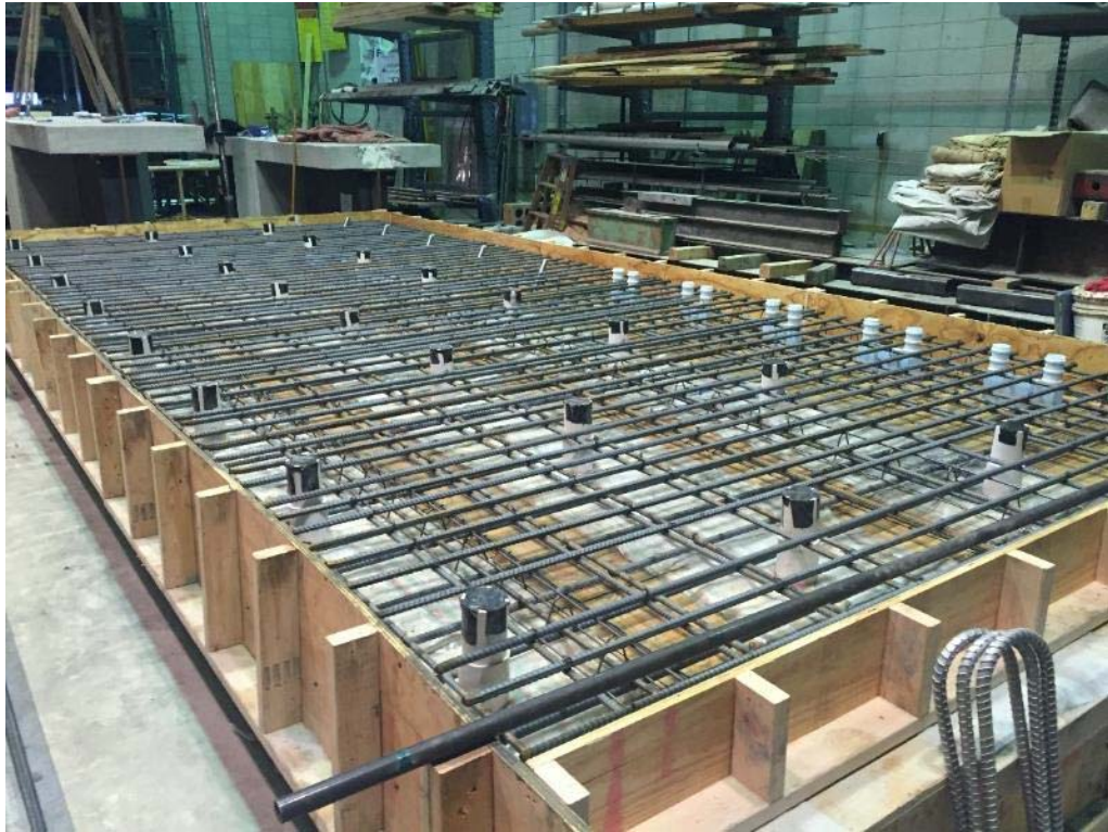
Figure 16 Bridge Deck Prior to Concrete Pour
