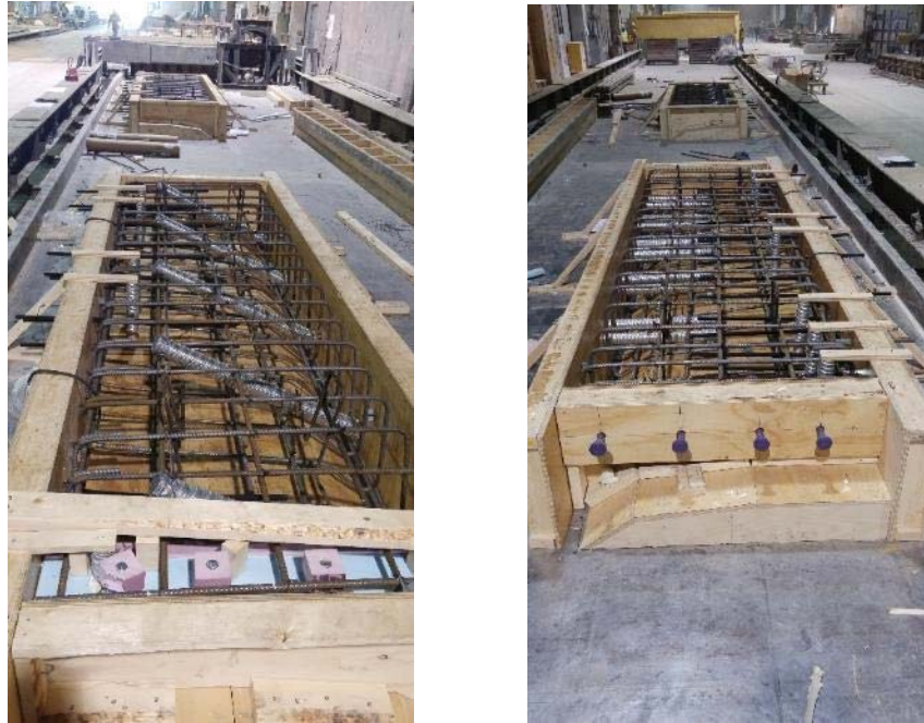
Figure 13 Precast Barrier Fabrication
