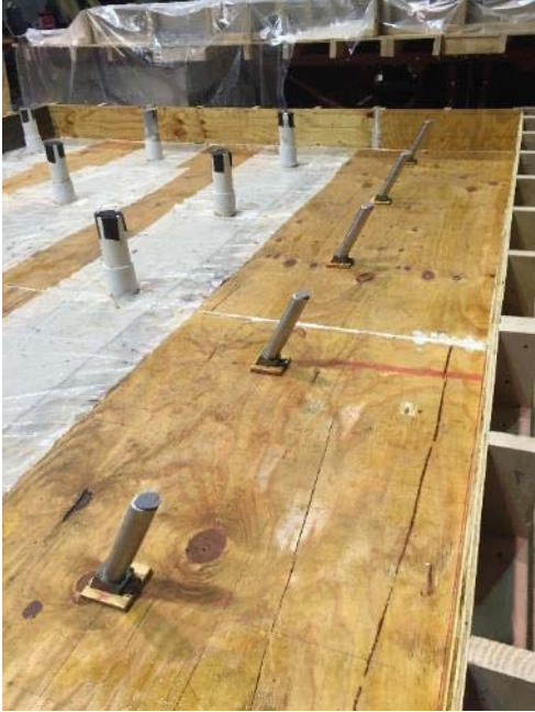
Figure 14 Inclined Bar Connection in Bridge Deck
