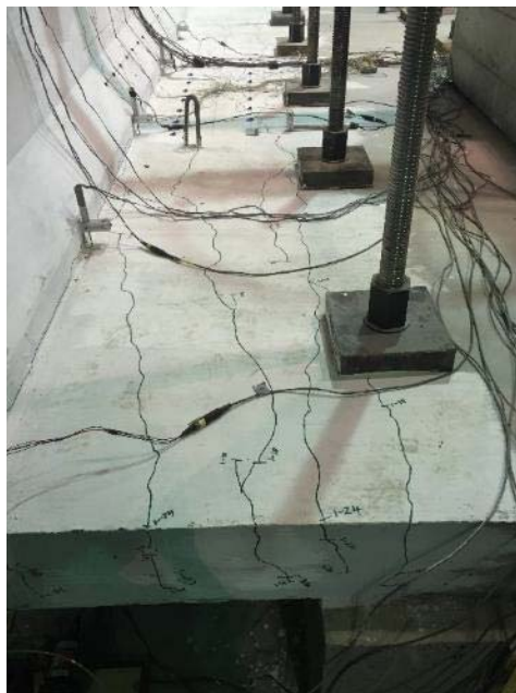
Figure 20 Test 1 (PBI Middle) Deck Cracks
