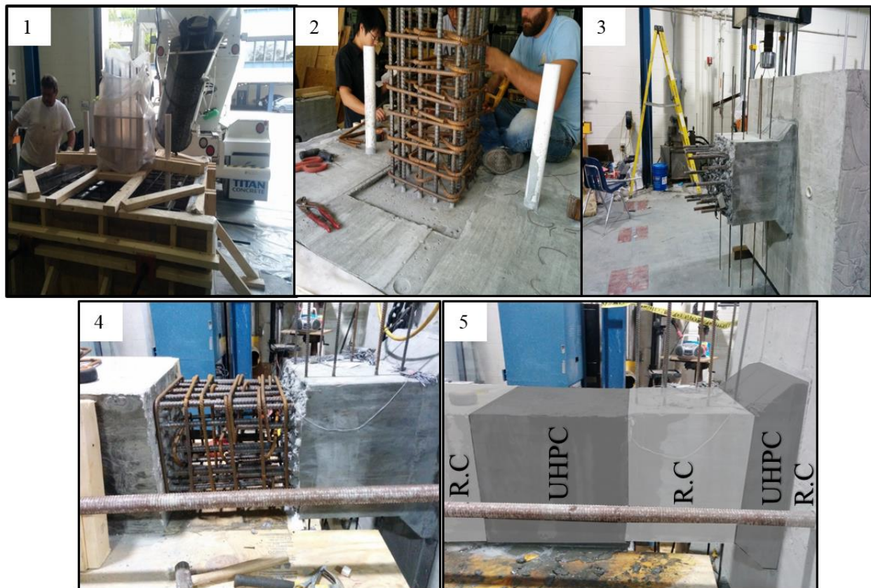
FIGURE 3 Specimen construction procedures.
