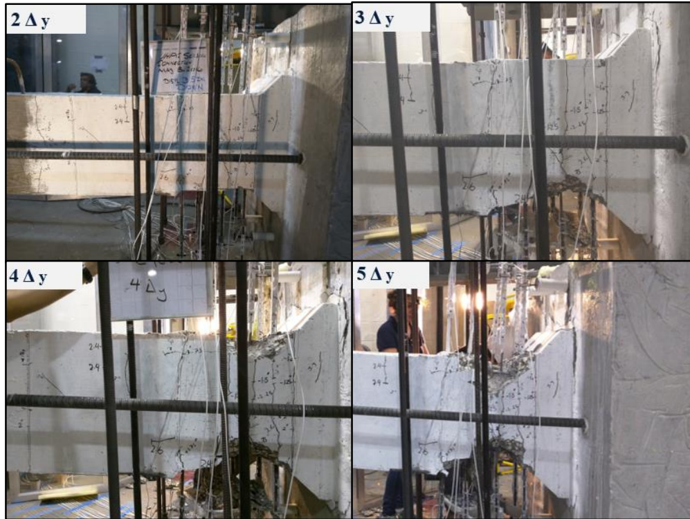
FIGURE 5 Plastic hinge damage at different displacement levels.
