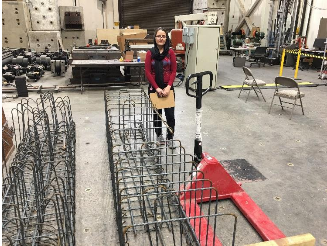
Fig. 43 – Cap beam reinforcement cage
