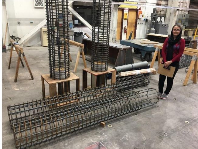
Fig. 43 – Column reinforcement cages
