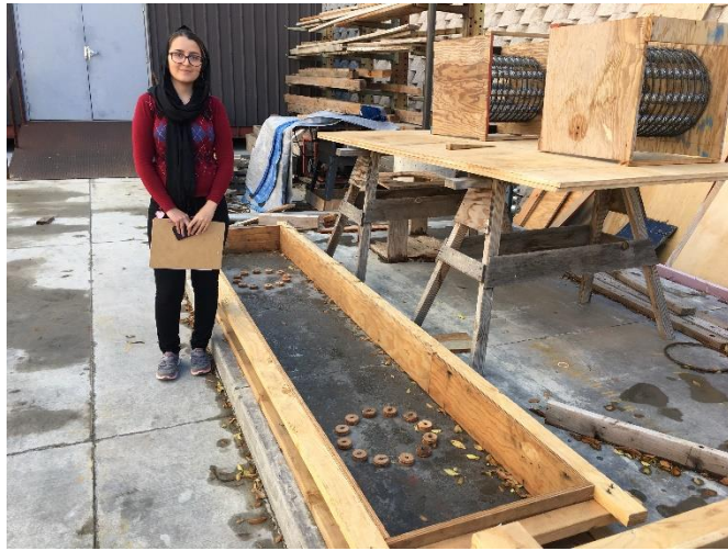
Fig. 41 – Formwork for the precast portion of cap beam
