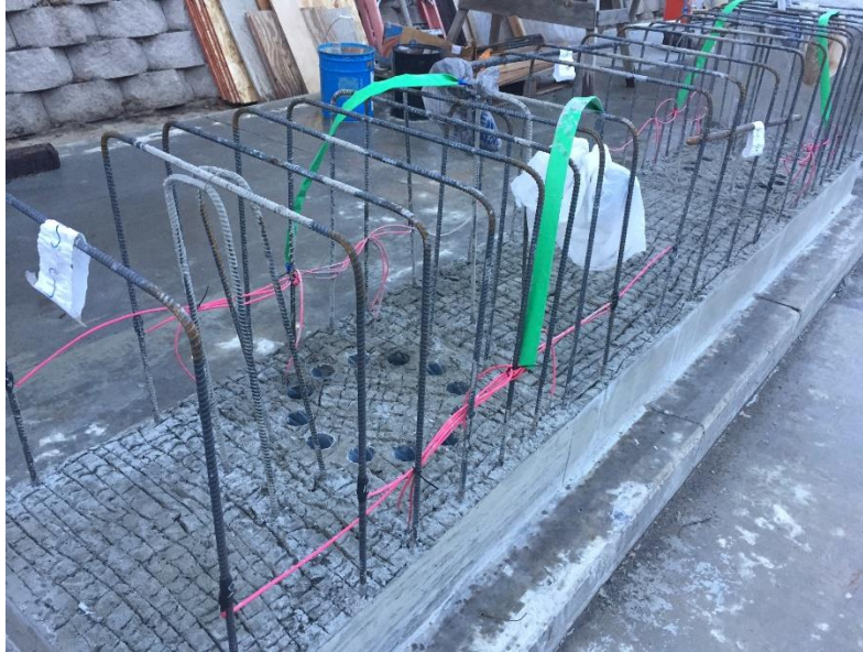
Fig. 47- Completed lower cap beam with corrugated ducts
