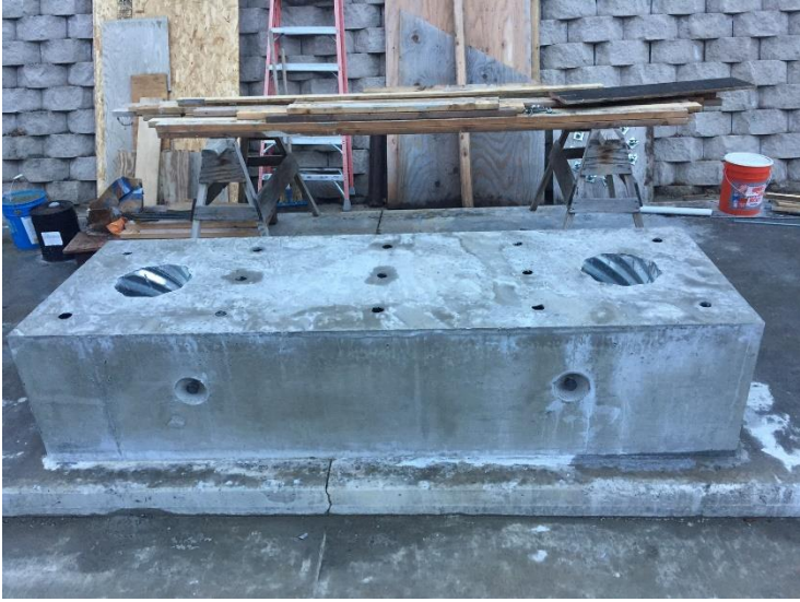
Fig. 45- Precast footing with sockets (pockets).
