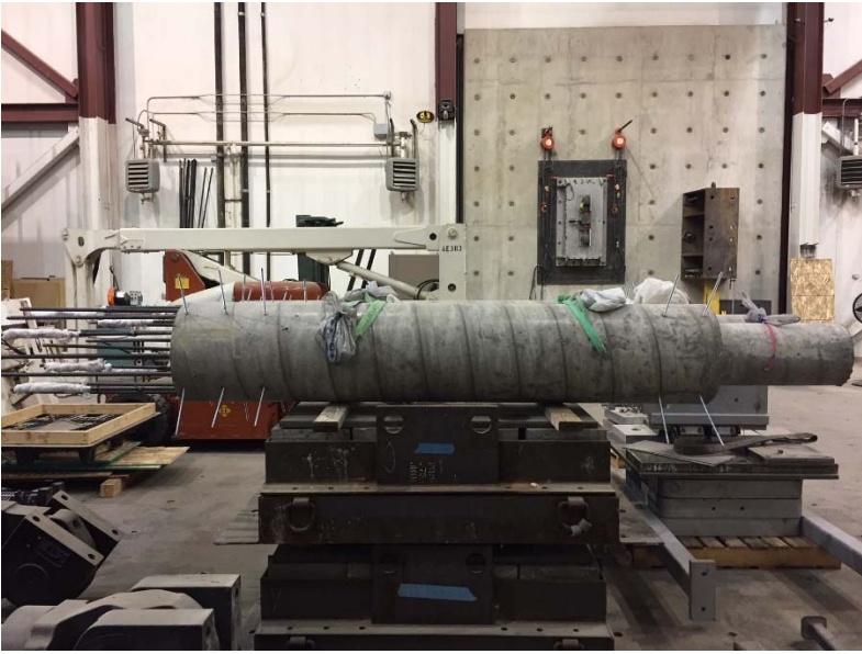
Fig. 46- Completed precast columns for the bent
