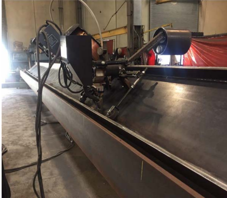
Fig. 52 –Welding of the flanges to the web
