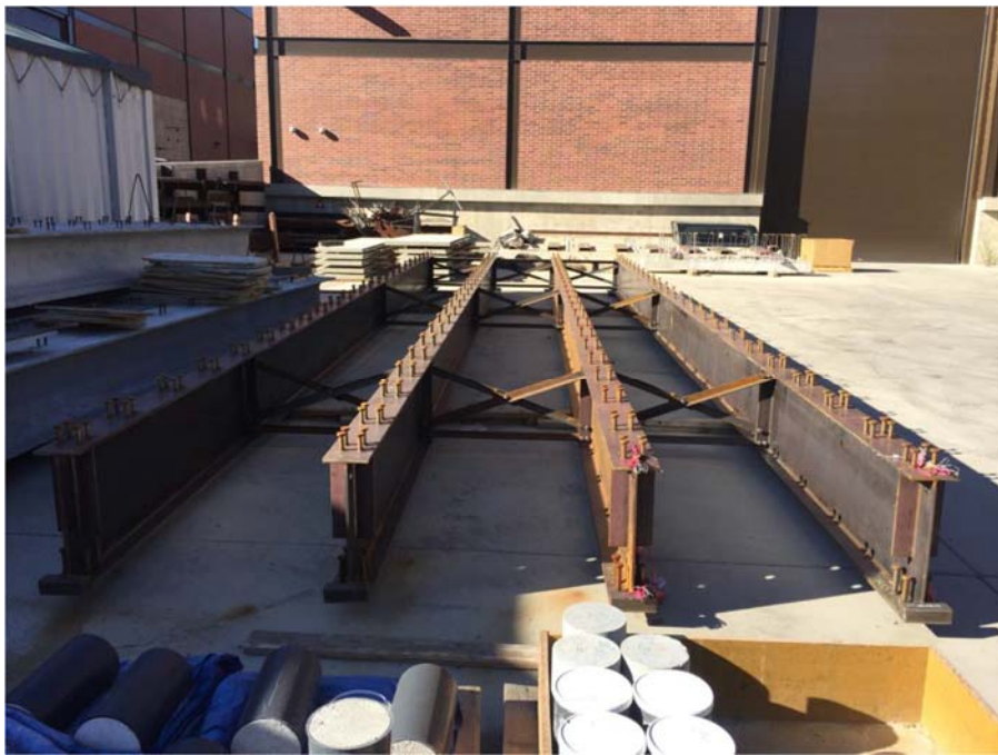
Fig. 55 –Assembled girders with cross braces
