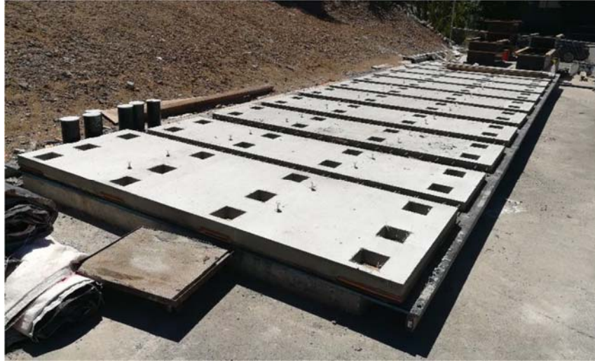
Fig. 50 –Completed deck panels for one of the spans
