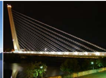
Puente del Alamillo By Santiago Calatrava
