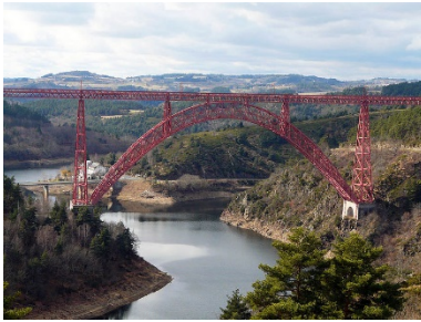
Garabit Viaduct By Gustave Eiffel
