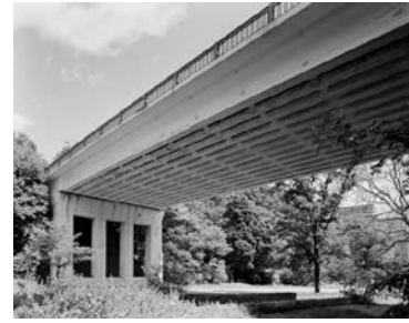
Walnut Lane Memorial Bridge By Gustave Magnel
