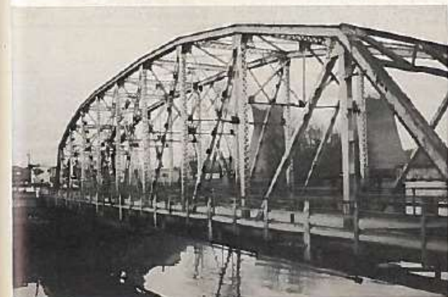
The Pocahontas Bridge is a truss structure, built in 1922
