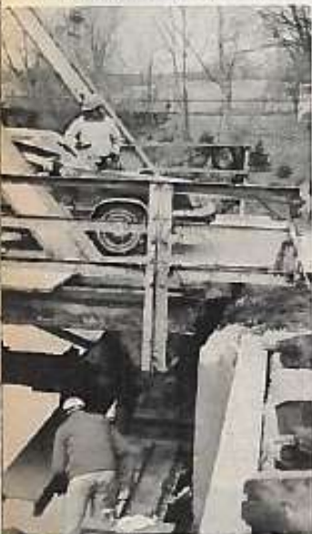
Jacking and bridge movement took place under traffic.
