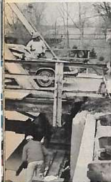
Jacking and bridge movement took place under traffic.
