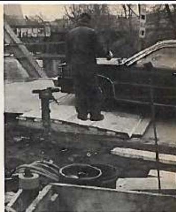
Temporary wooden ramps were used for traffic during the move.
