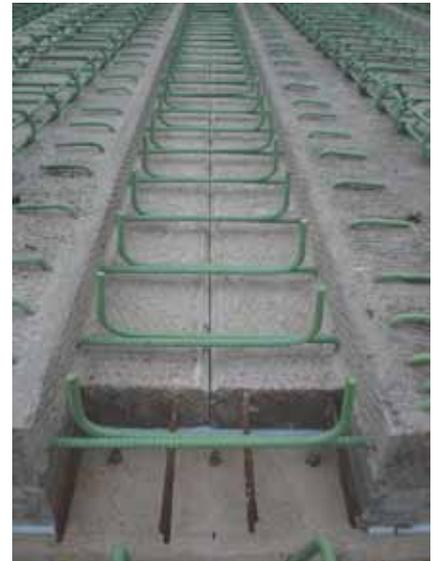
View of a longitudinal joint between precast sections before installing field-placed reinforcement.
