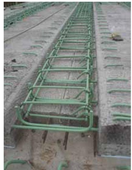
View of a longitudinal joint after the placement of the “drop-in” reinforcing cage.
