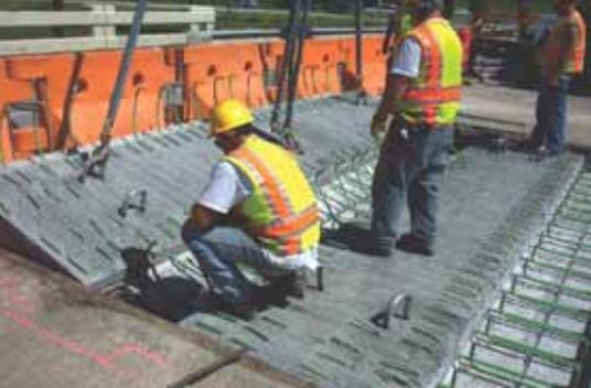
A precast concrete section being lowered into place adjacent to another during the rehabilitation of Bridge 6679.
