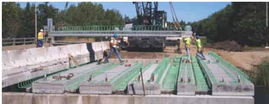
On Bridge 04002, a precast concrete beam is being moved into place alongside five sections that have already been erected. The typical 6 ft 0 in. beam width can be changed to accommodate bridge width.
