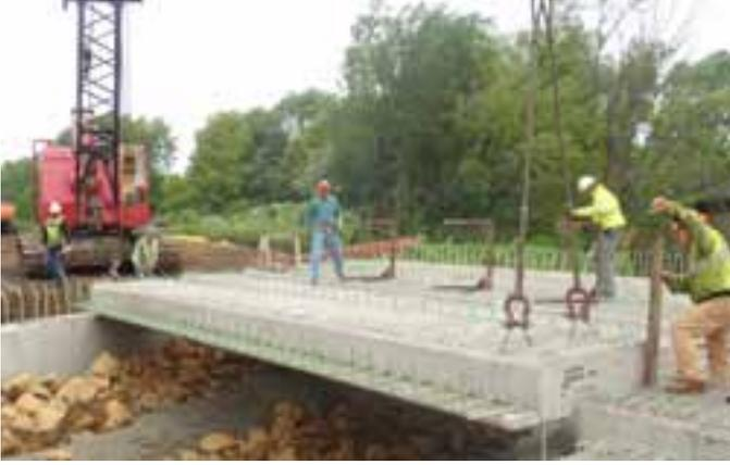
At Bridge 66004, a precast concrete beam is lowered onto the substructures. The diamond pattern in the concrete provided a roughened surface to assist with composite action. Presently, a roughened surface is provided on all contact surfaces except the tops of the flanges.
