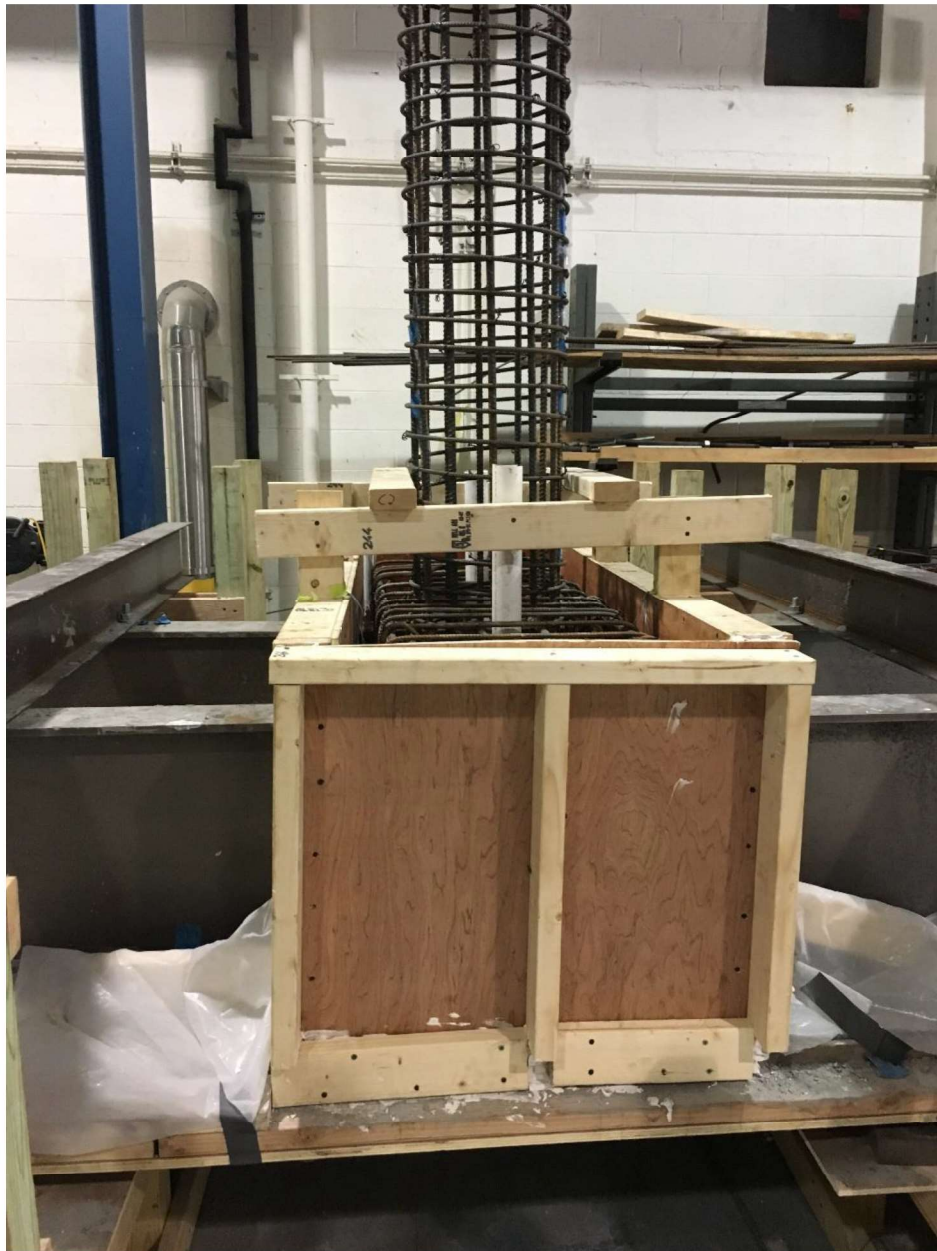
Figure 3-25 Formworks for step 2 of construction.
