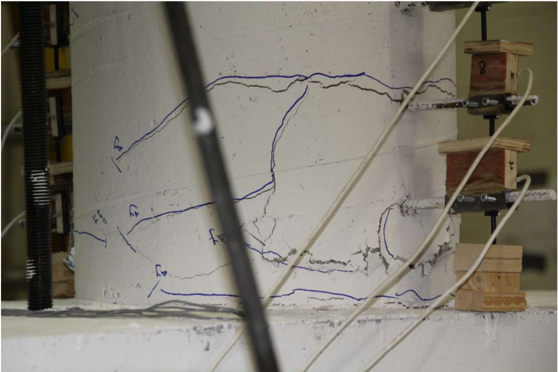
Figure 4-4 Crushing of concrete on the North side of the column at 1\Delta_y .
