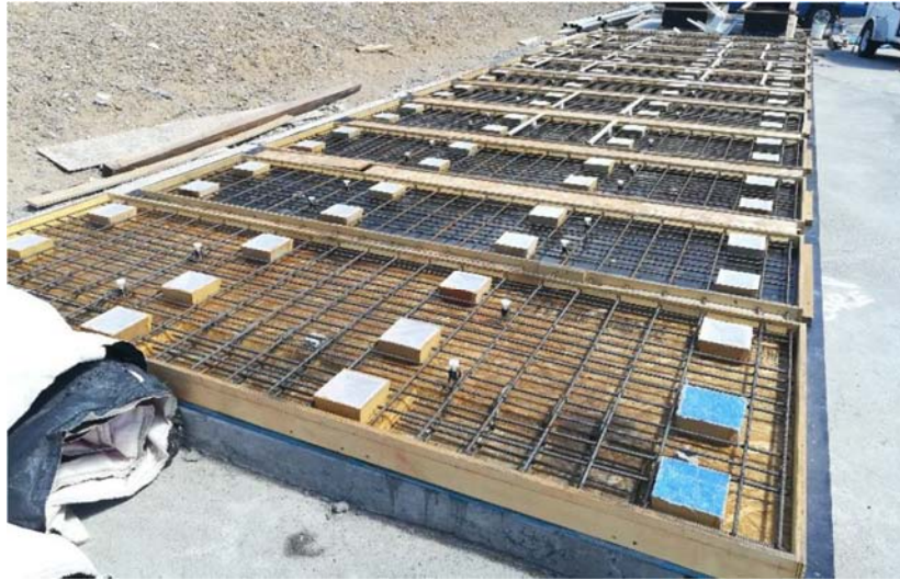
Fig. 49 –Deck panel steel reinforcement
