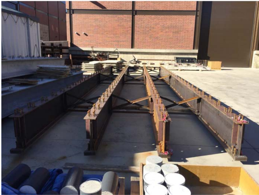
Fig. 55 –Assembled girders with cross braces
