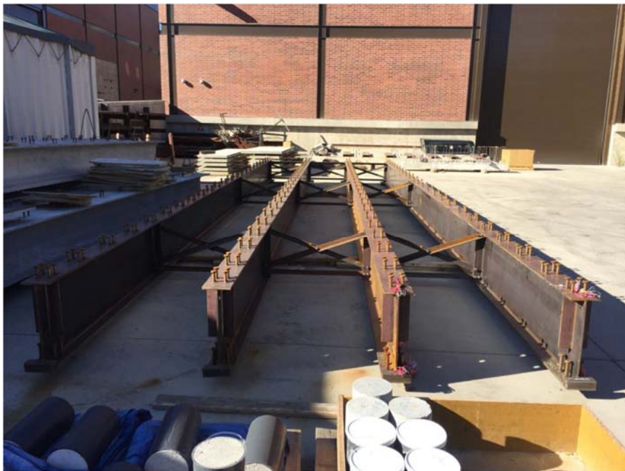
Fig. 55 –Assembled girders with cross braces
