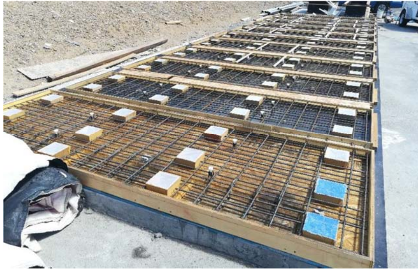
Fig. 49 –Deck panel steel reinforcement
