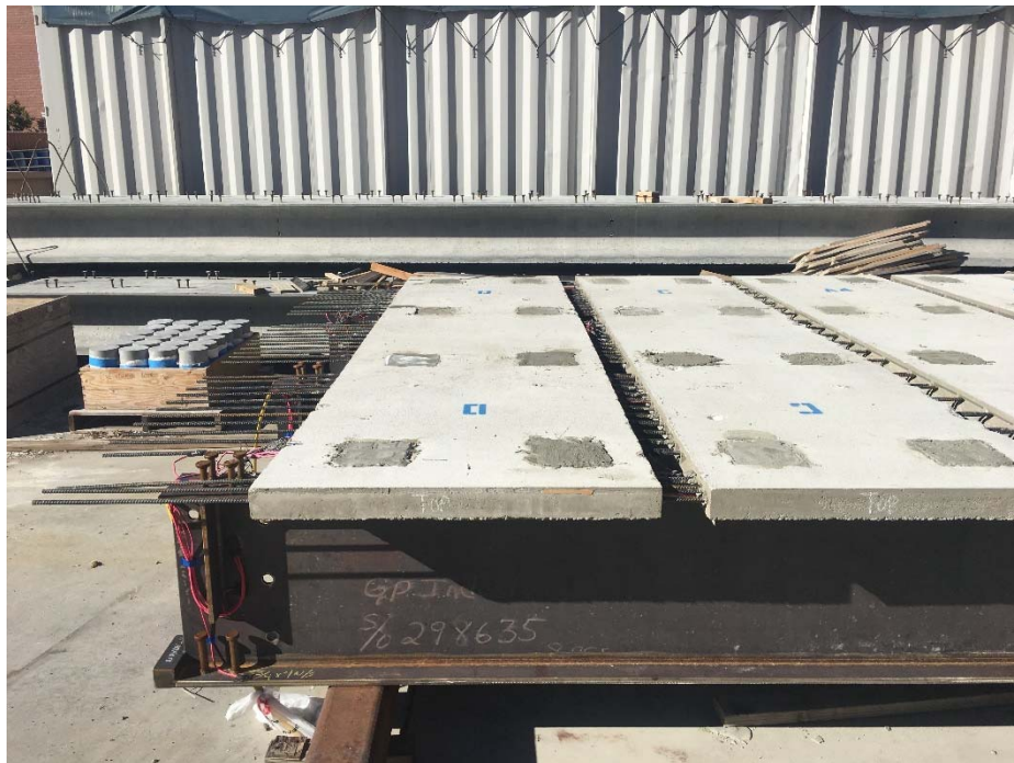
Fig. 57- Grouted deck pockets
