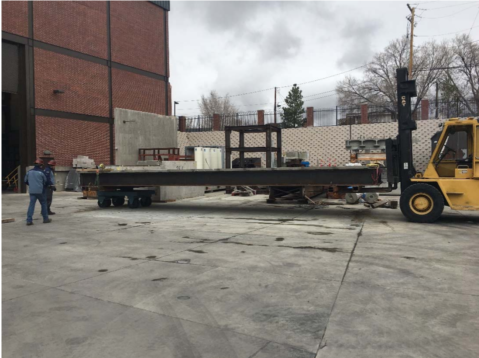
Fig. 59- Moving complete span to lab
