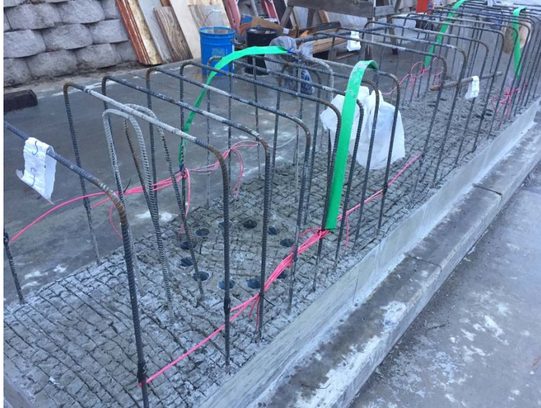
Fig. 47- Completed lower cap beam with corrugated ducts
