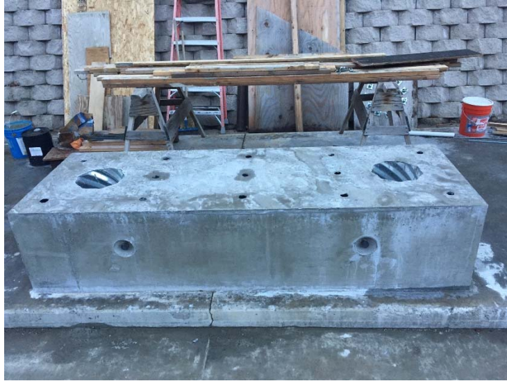
Fig. 45- Precast footing with sockets (pockets).
