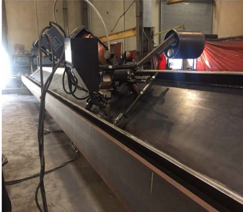
Fig. 52 –Welding of the flanges to the web
