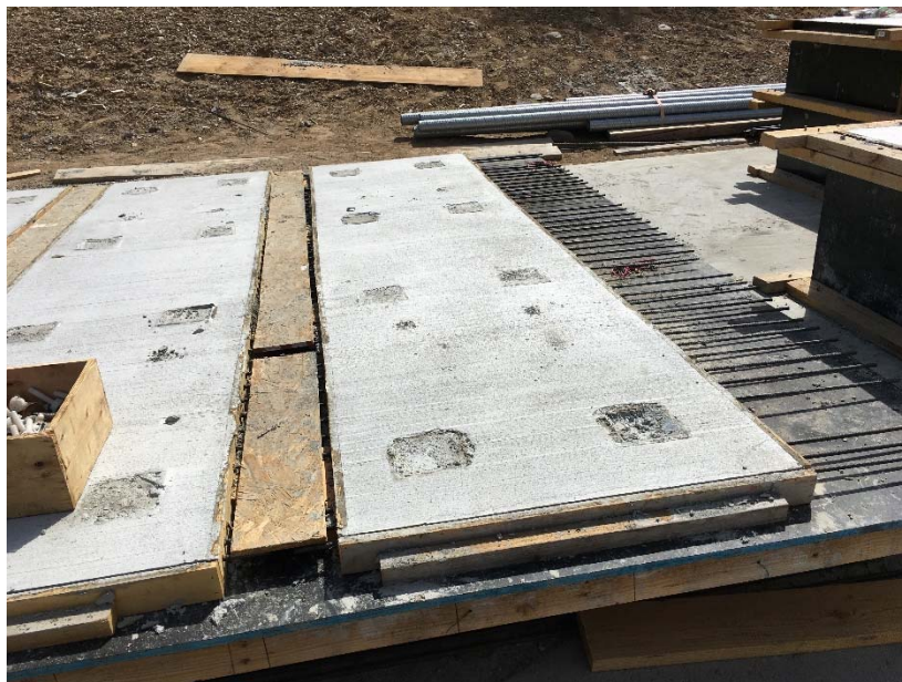
Fig. 51 –Edge deck panel with extended reinforcement on the right
