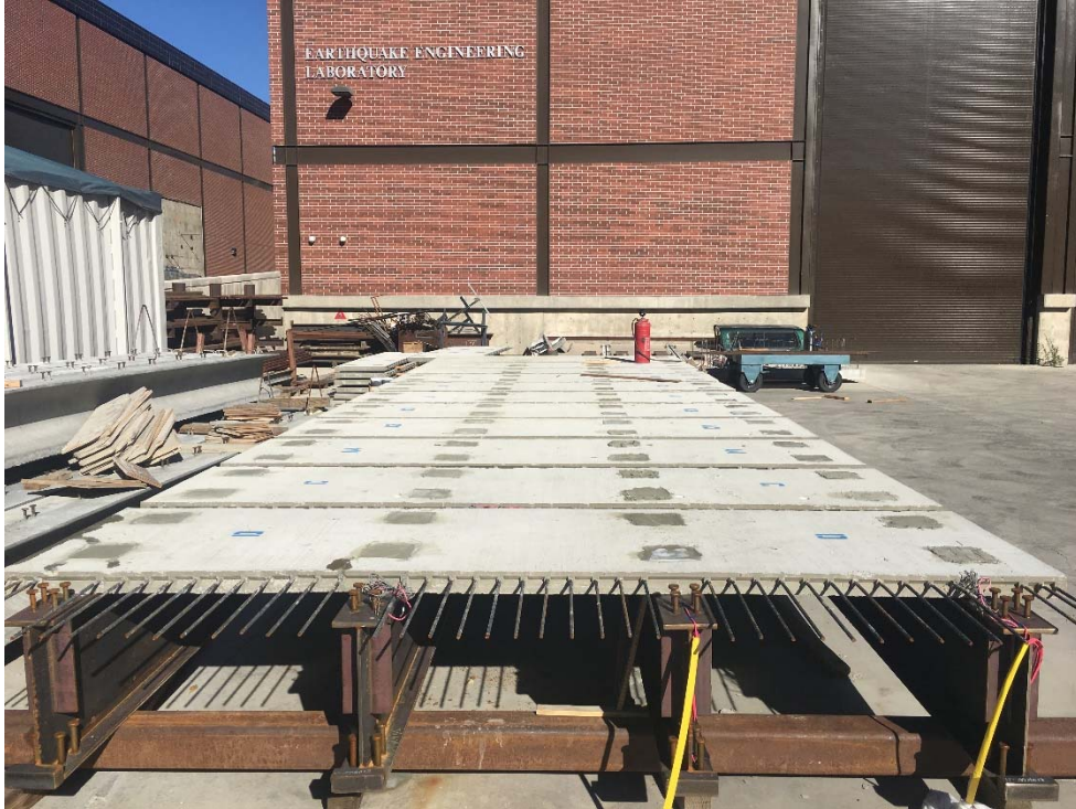
Fig. 56- End view of superstructure after placing and grouting of pockets
