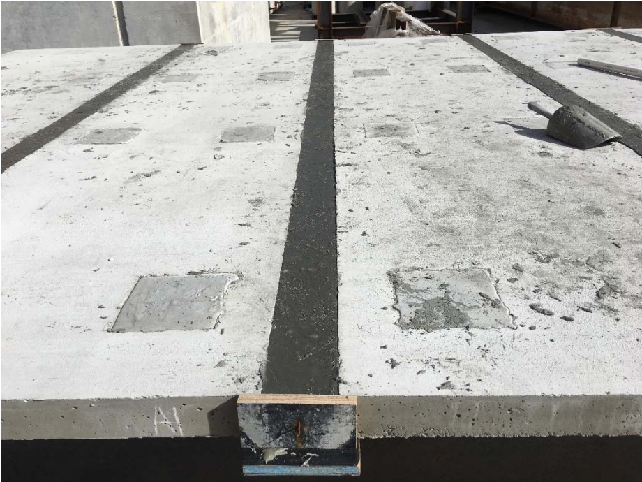
Fig. 58- UHPC in deck joints
