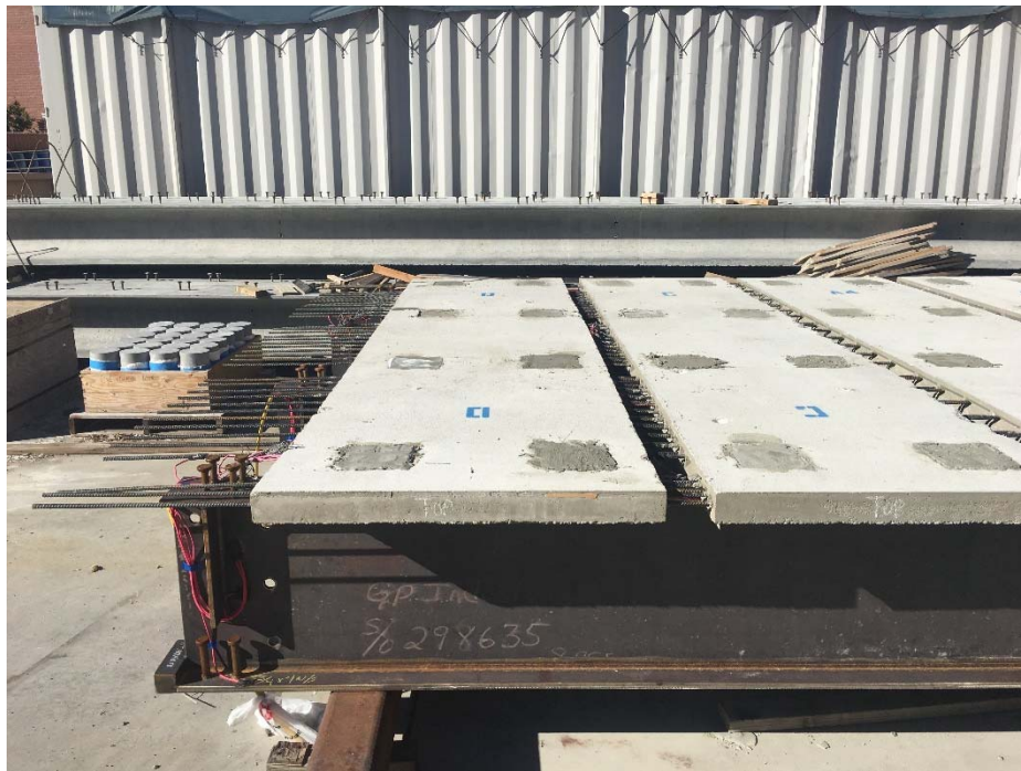
Fig. 57- Grouted deck pockets
