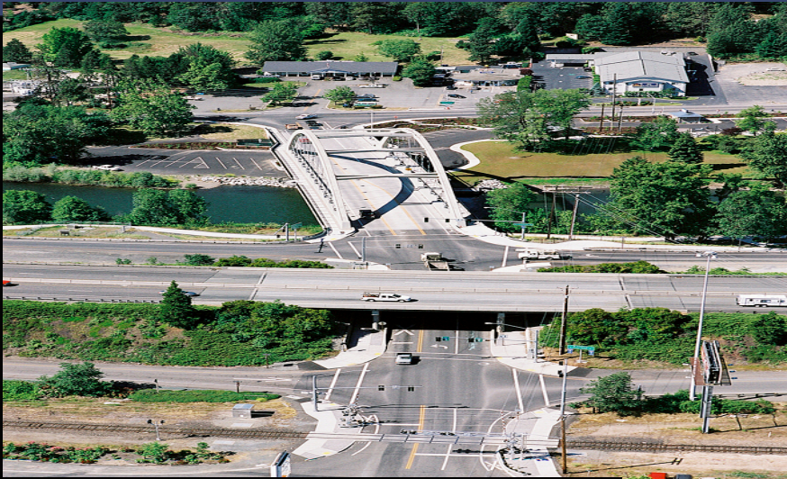
5 day closure to slide bridge into place
