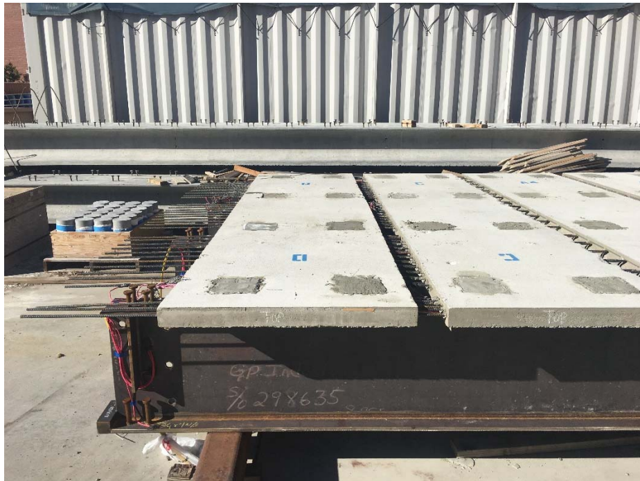
Fig. 57 – Grouted deck pockets
