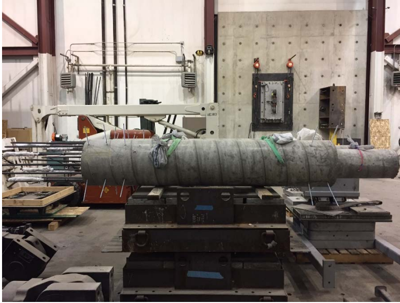
Fig. 46 – Completed precast columns for the bent
