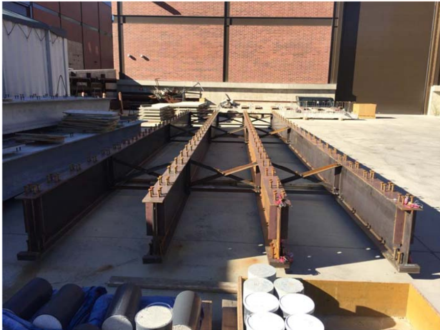
Fig. 55 – Assembled girders with cross braces
