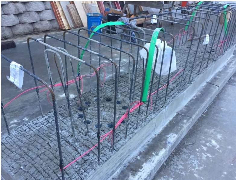
Fig. 47 – Completed lower cap beam with corrugated ducts
