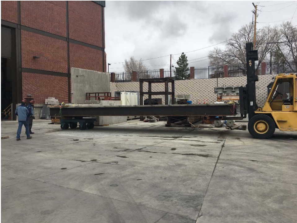
Fig. 59 – Moving complete span to lab
