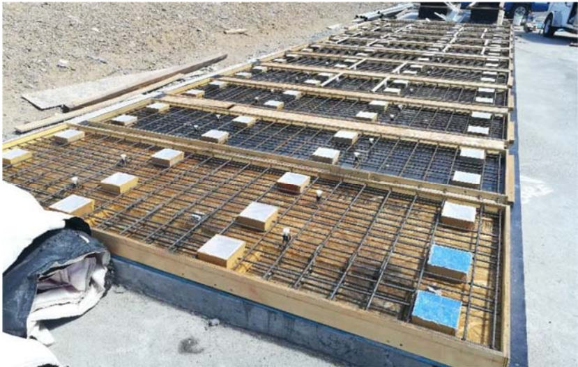
Fig. 49 – Deck panel steel reinforcement
