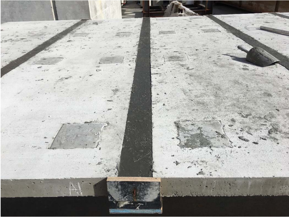
Fig. 58 – UHPC in deck joints
