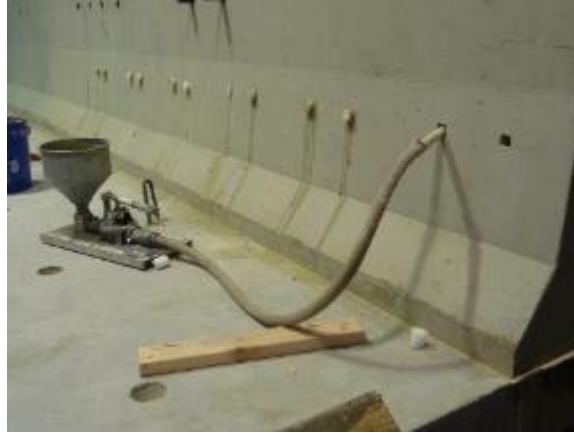
Figure 4.22. Grouting of U-bar pockets
