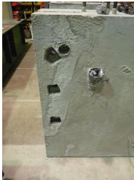
Figure 4.16. Pockets used to install transverse barrier-to-barrier connection
