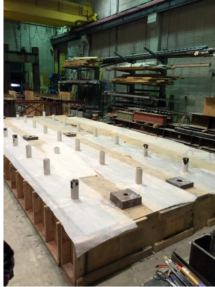
Figure 4.5. Bridge deck supporting beams with formwork
