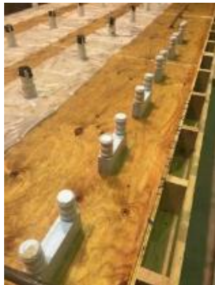
Figure 4.8. Deck block outs to facilitate U-bar installation
