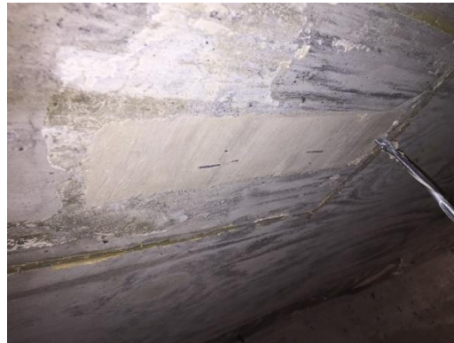
Figure 4.23. Finished U-bar grout pocket
