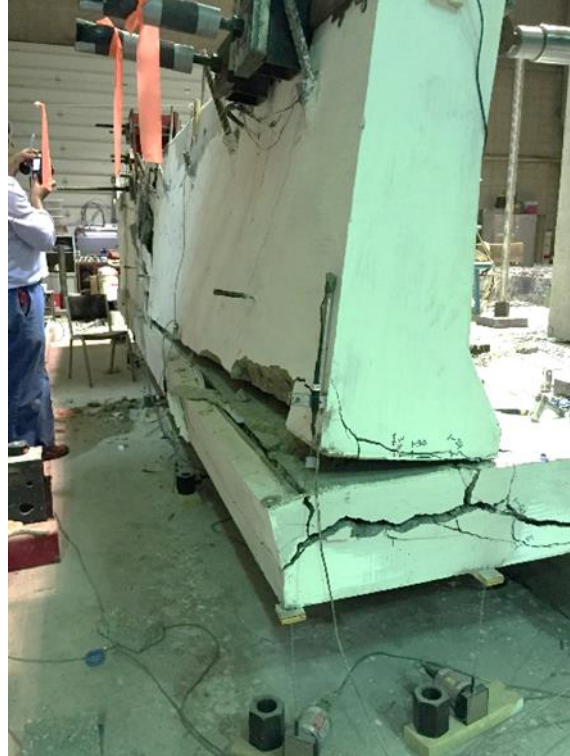
Figure 5.34. Damage to barrier and deck after Test 5 pull test
