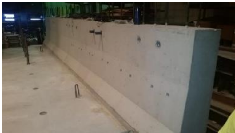
Figure 4.24. Completed barrier installation
