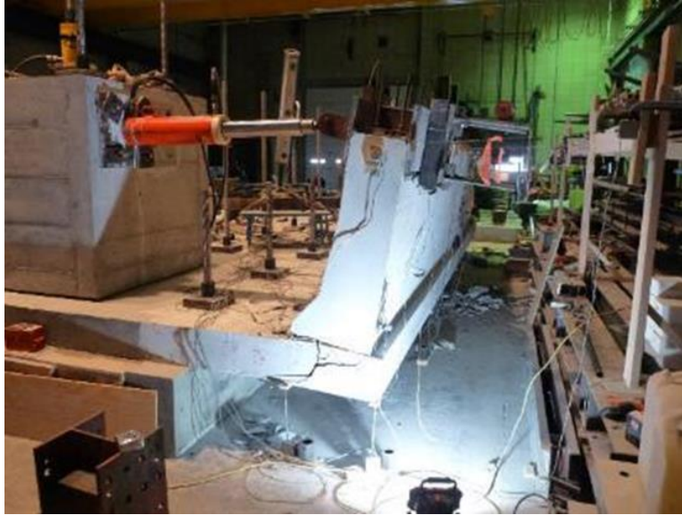
Figure 5.40. Final barrier deflection and the corresponding damage to the bridge deck during Test 5
