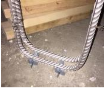
Figure 4.17. Reinforcing steel bar chairs for #5 bars
