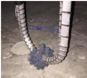
Figure 4.18. Reinforcing steel bar chairs for #7 bars
