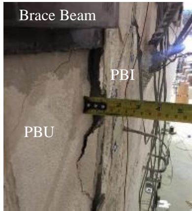
Figure 5.29. Difference in barrier movement at barrier-to-barrier connection at the maximum load during Test 4
