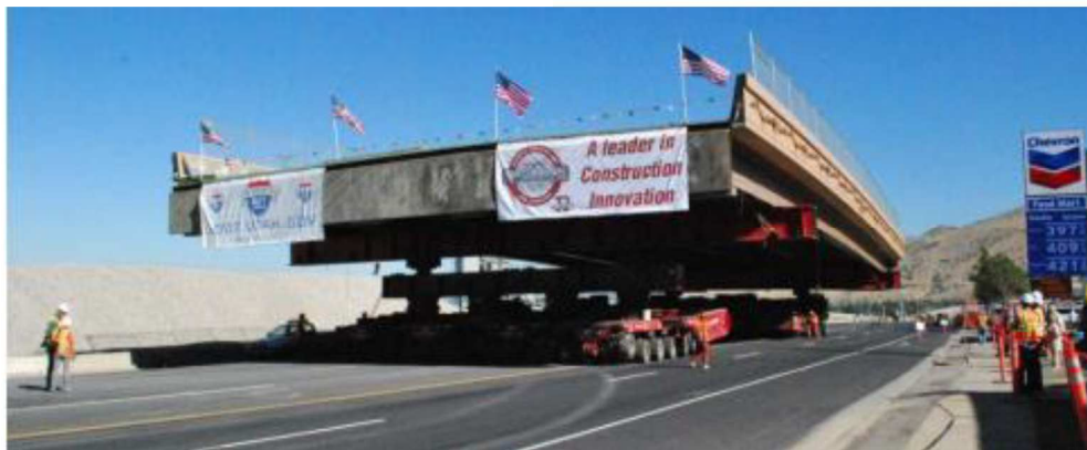
Figure 1: ABC superstructure positioning [5]
