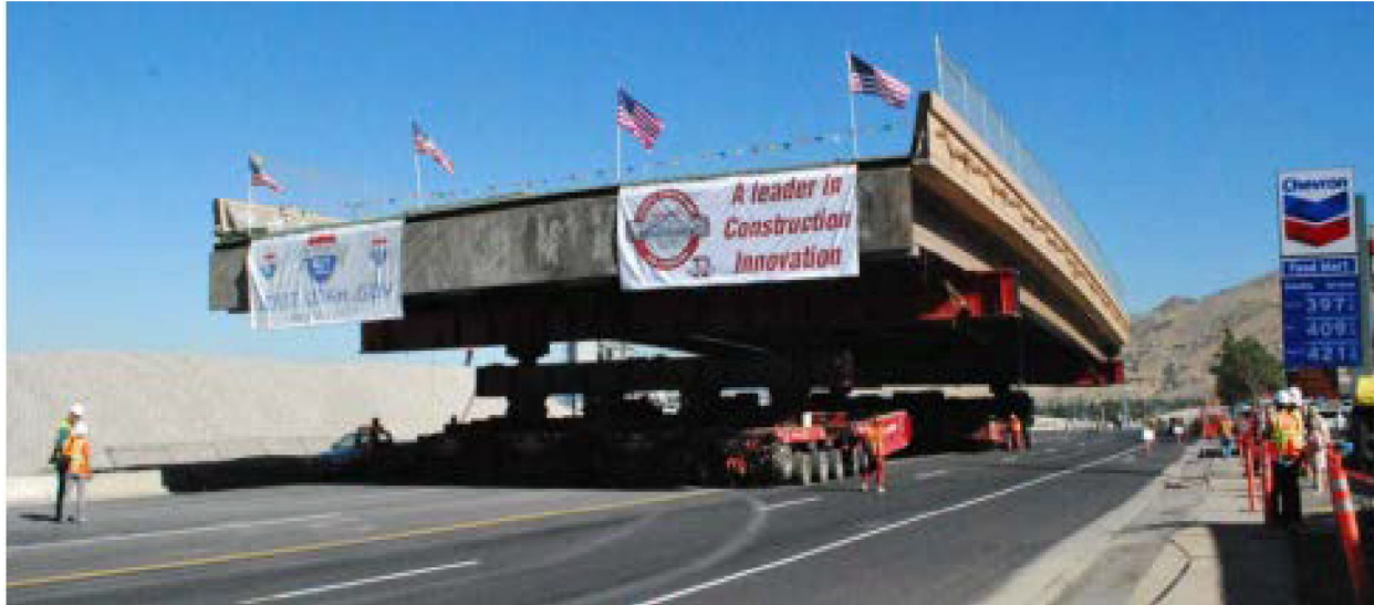
Figure 1: ABC superstructure positioning [5]
