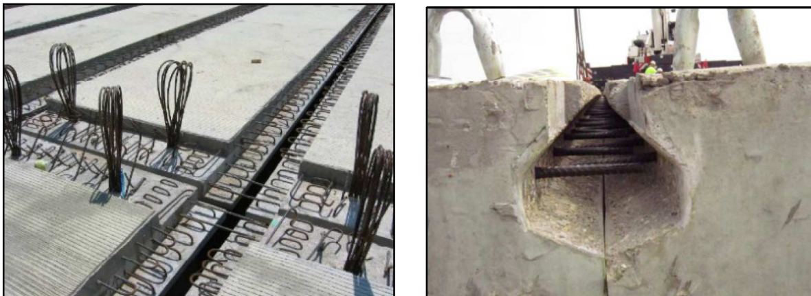
Figure 2: Examples of various types of ABC closure joints [6]–[9]
