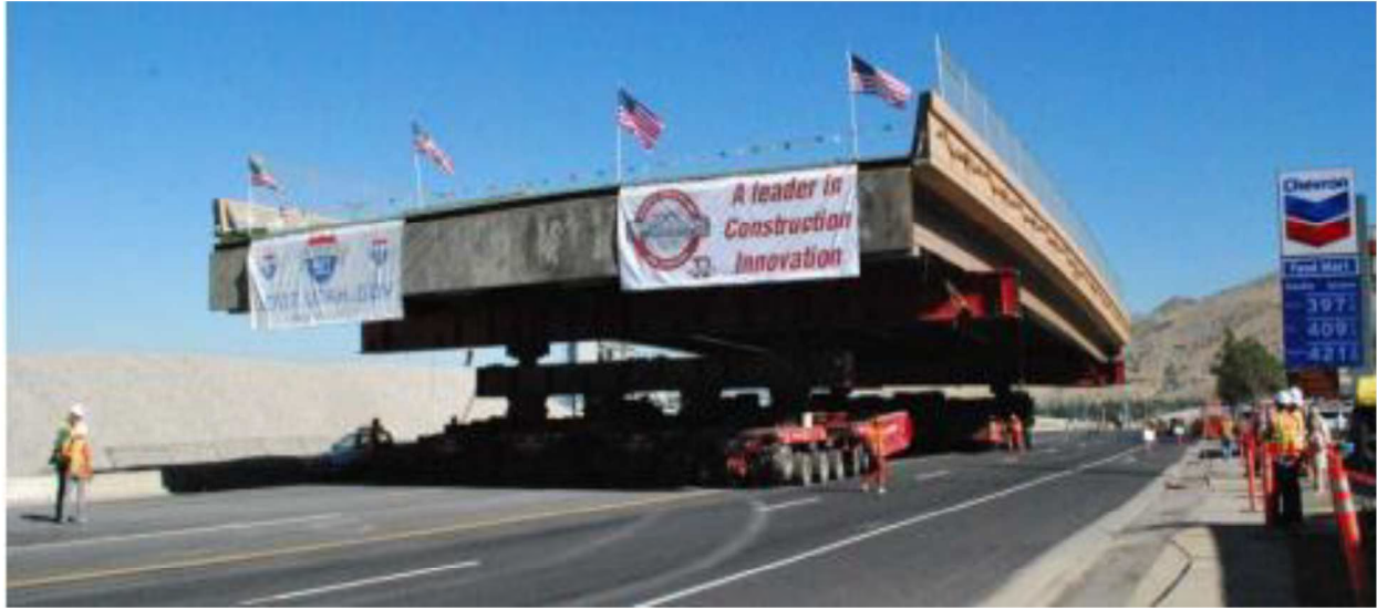
Figure 1: ABC superstructure positioning [5]
