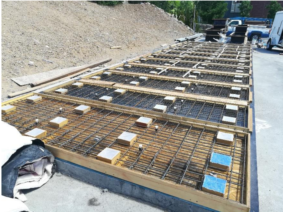
Figure A.40 Formwork and reinforcement of deck panels
