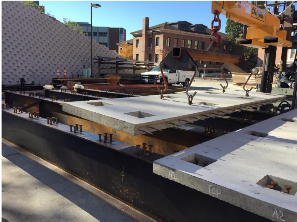
Figure A.42 Placing deck panels on the girders
