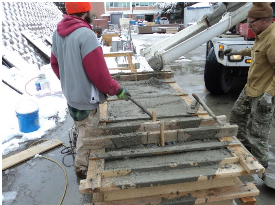
Figure A.28 Casting and vibration of footing concrete
