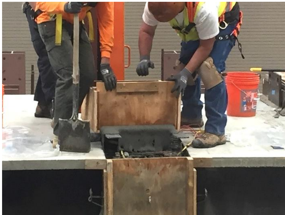
Figure A.50 Casting UHPC in the top layer of cap beam
