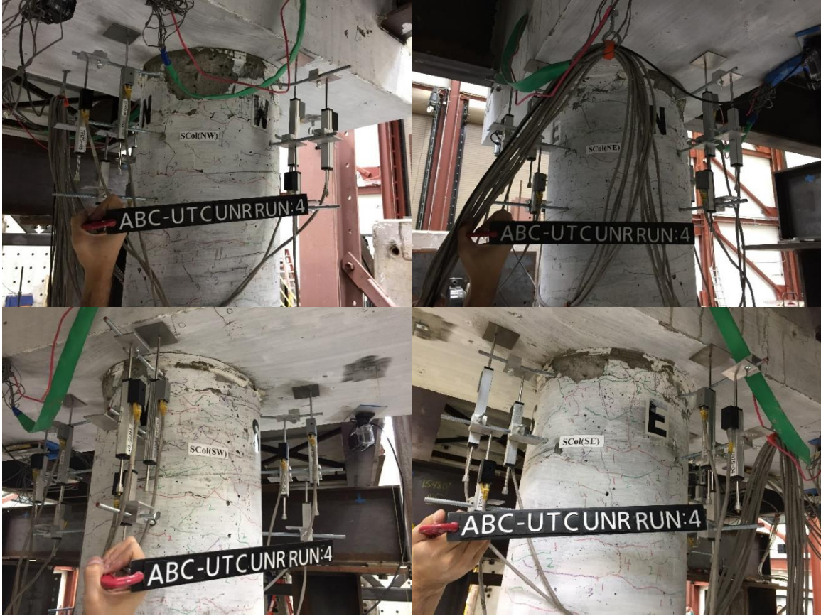
Figure B.5 Damage states of the south column plastic hinges after Run 4
