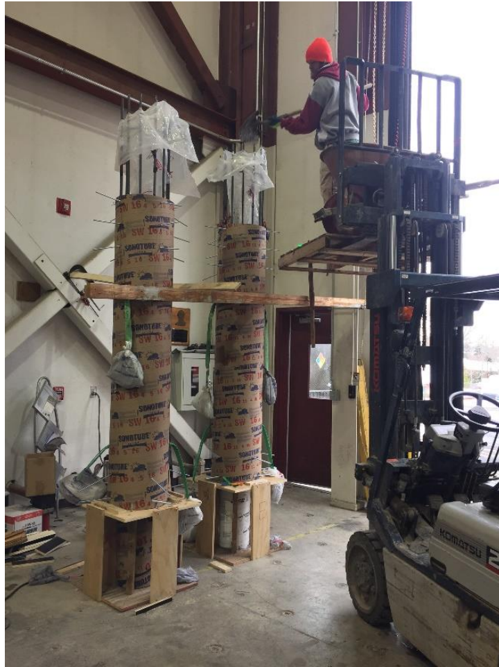
Figure A.34 Casting the column concrete
