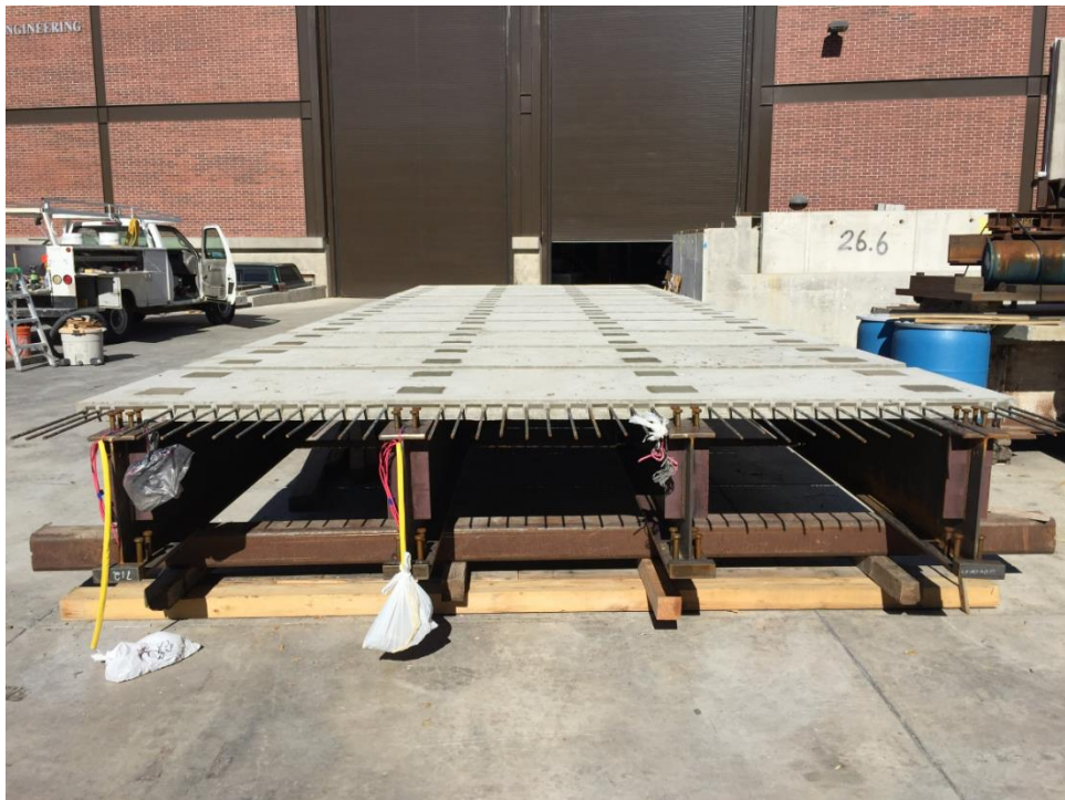
Figure A.45 Superstructure after casting grout and UHPC in deck pockets
