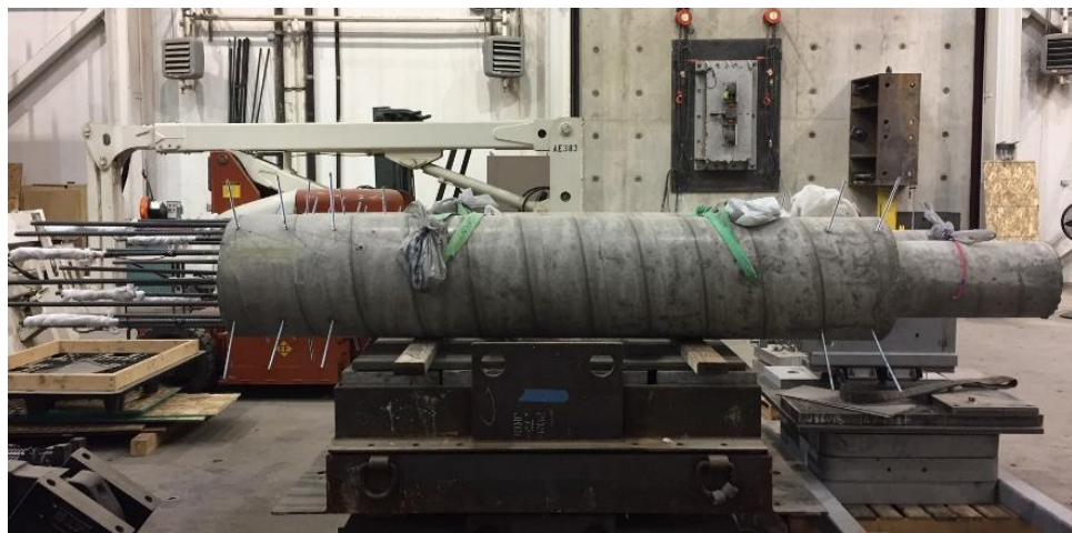
Figure A.35 Columns after casting the concrete
