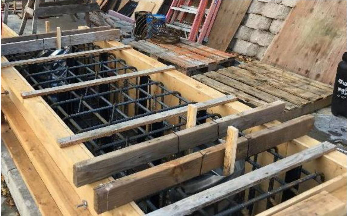
Figure A.27 Footing reinforcement, formwork, PVC ducts, and corrugated pipes
