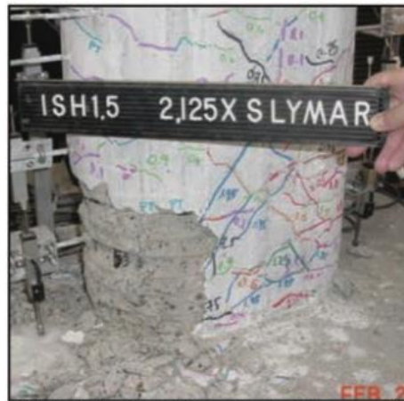
DS-4: lateral and longitudinal bars visible
