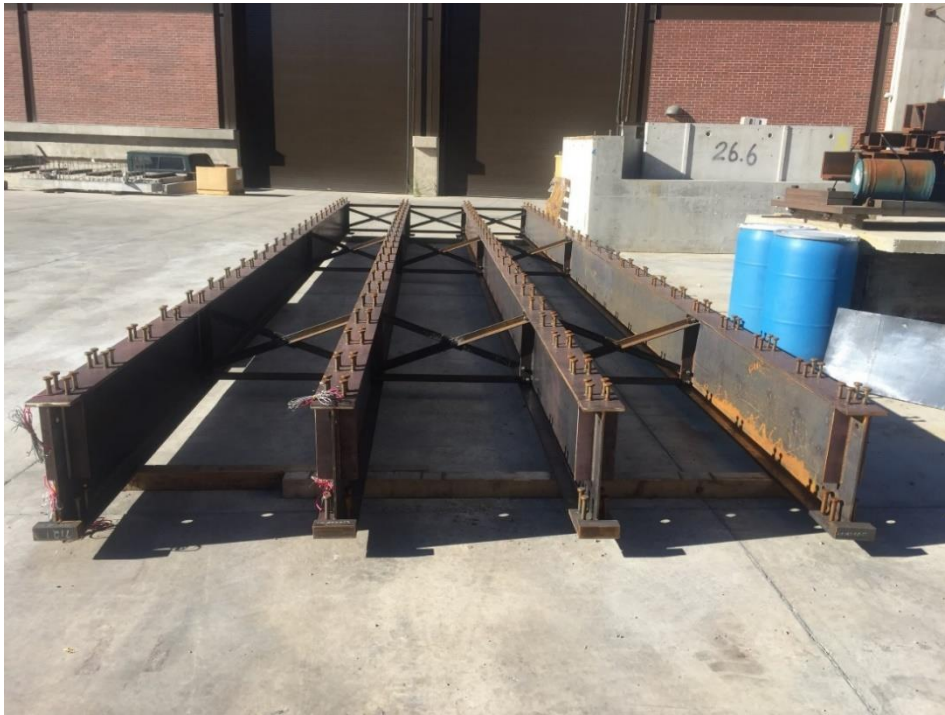
Figure A.26 Assembled girders and cross frames (east span)
