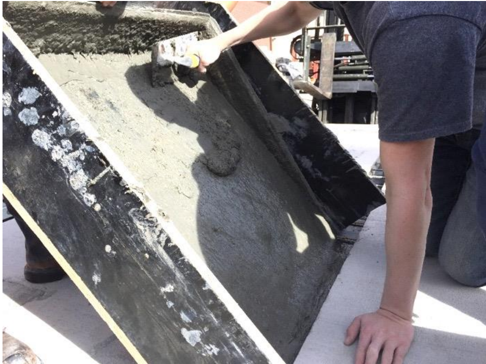
Figure A.44 Casting UHPC in the deck panels joints
