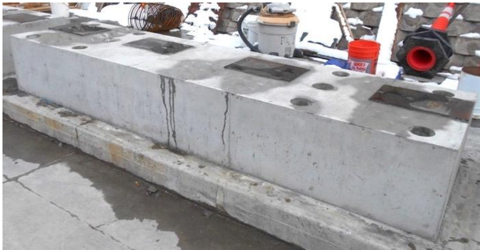
Figure A.47 Superstructure after casting grout and UHPC in deck pockets
