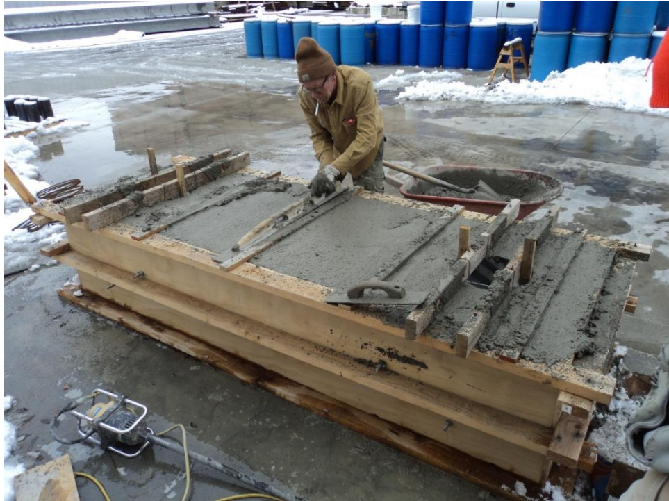
Figure A.29 Finishing the footing concrete surface
