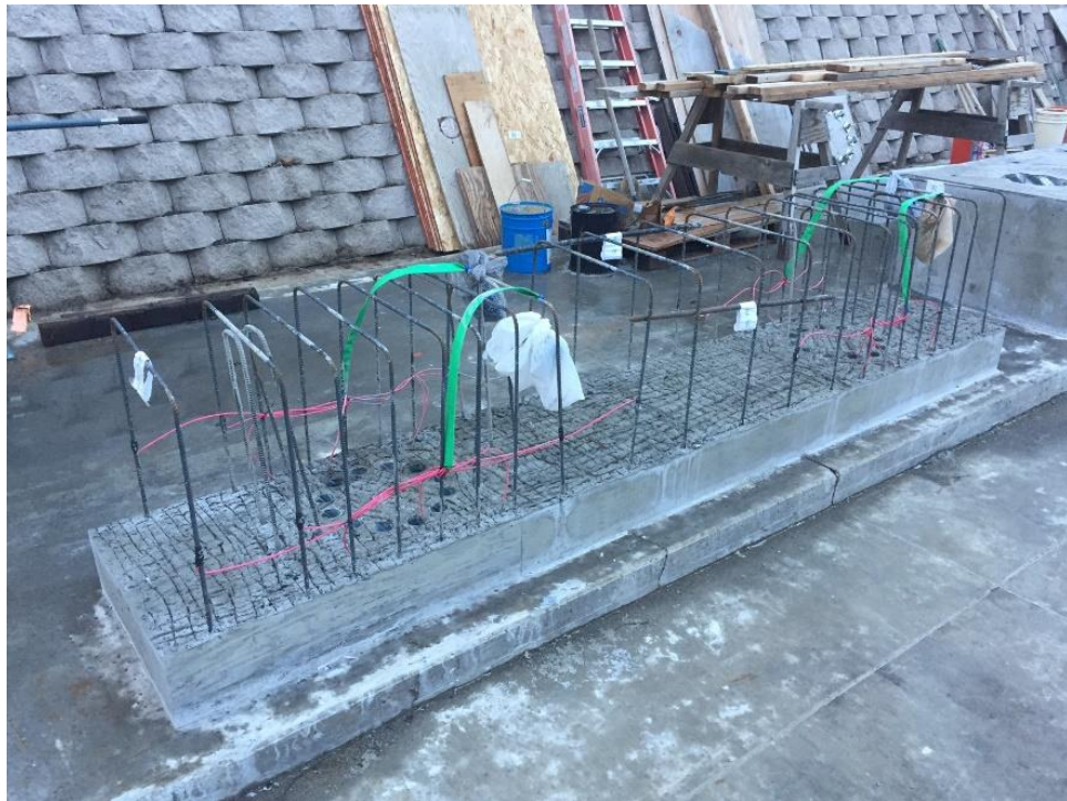
Figure A.39 Cap beam after casting and removing the formwork
