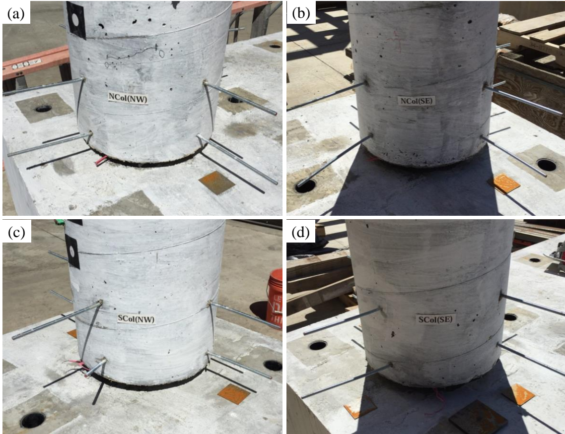
Figure 3.18 Damage states of the rebar hinge after Run 8: (a) North column - Northwest view, (b) North column - Southeast view, (c) South column - Northwest view, (d) South column - Southeast view (Images by Elmira Shoushtari)
