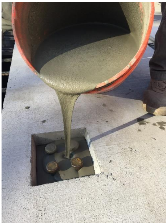
Figure A.43 Pouring grout in pockets of deck panels
