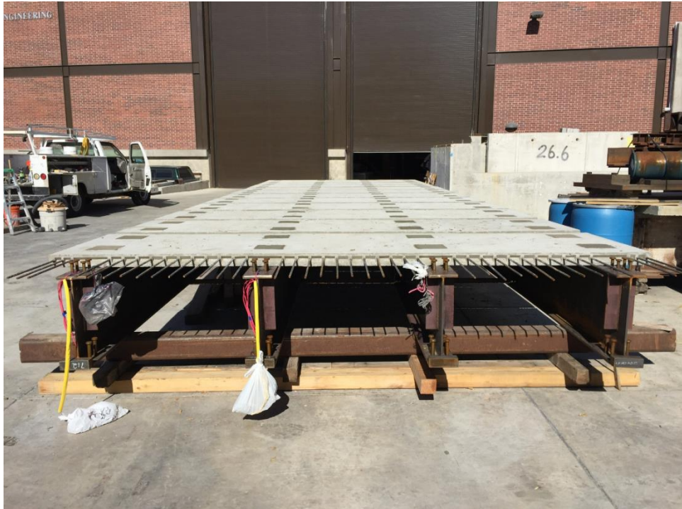
Figure A.46 Superstructure after casting grout and UHPC in deck pockets
