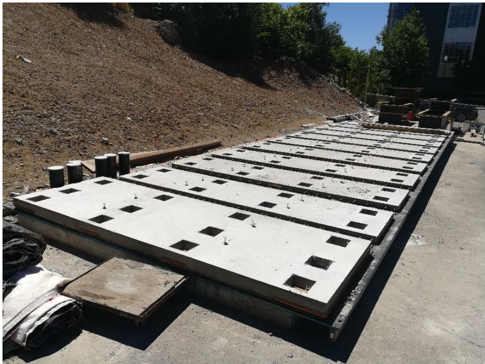
Figure A.41 Deck panels after removing the formwork
