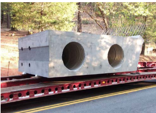
Fig. 3 – Precast abutment segments for Fort Goff Creek bridge in California (photos are courtesy of Dorie Mellon as adopted from Caltrans ABC-UTC seminar)
