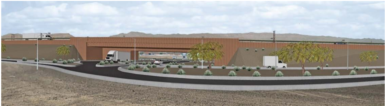
Fig. 2 – I-15 / US 93 Garnet Interchange ABC bridge in Las Vegas, NV completed in Dec 2018
