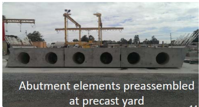
Fig. 3 – Precast abutment segments for Fort Goff Creek bridge in California (photos are courtesy of Dorie Mellon as adopted from Caltrans ABC-UTC seminar)
