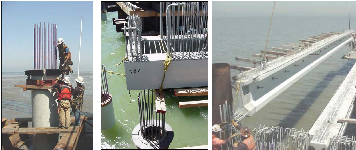
Fig. 1 – San Mateo-Hayward Bridge Widening Project in California using prefabricated elements (courtesy of Caltrans ABC pilot program, Roberto Lacalle)
