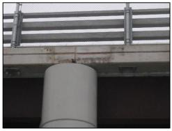
Fig.12: Installed UHPC Link Slab
