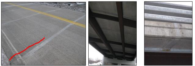
Fig. 19: Parallel Cracks to UHPC Connection Fig. 20: Bridge Deck Underside Fig 21: Transverse Joint
