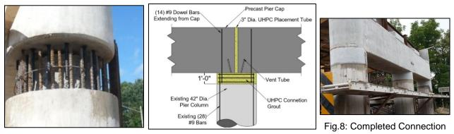
Fig. 6: Rebar Connection
