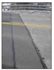
Fig. 23: North Abutment Expansion Joint
