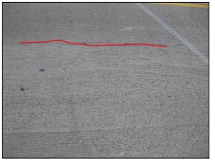
Fig. 22: Longitudinal Crack – Perpendicular to UHPC
