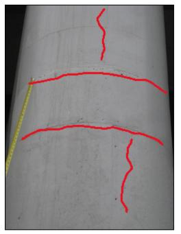
Fig. 10: Vertical Cracks in Column & Pier Cap
