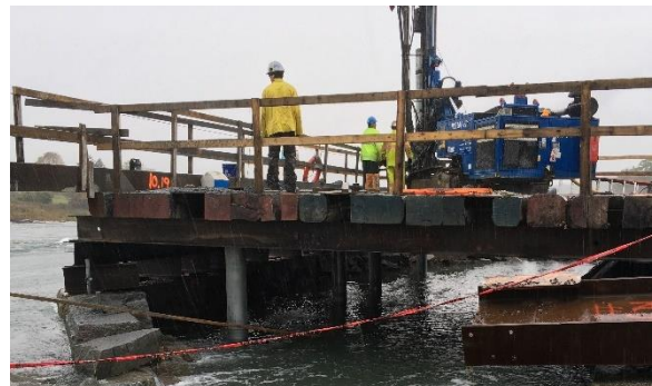
Figure 3 - Drilling Piles while staying out of the water
