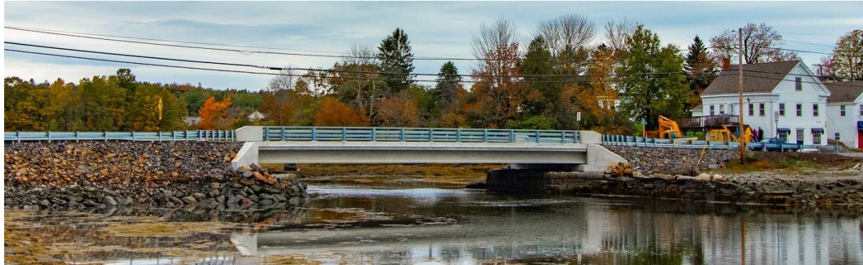
Figure 6 - Completed Bridge after 33-day Closure
