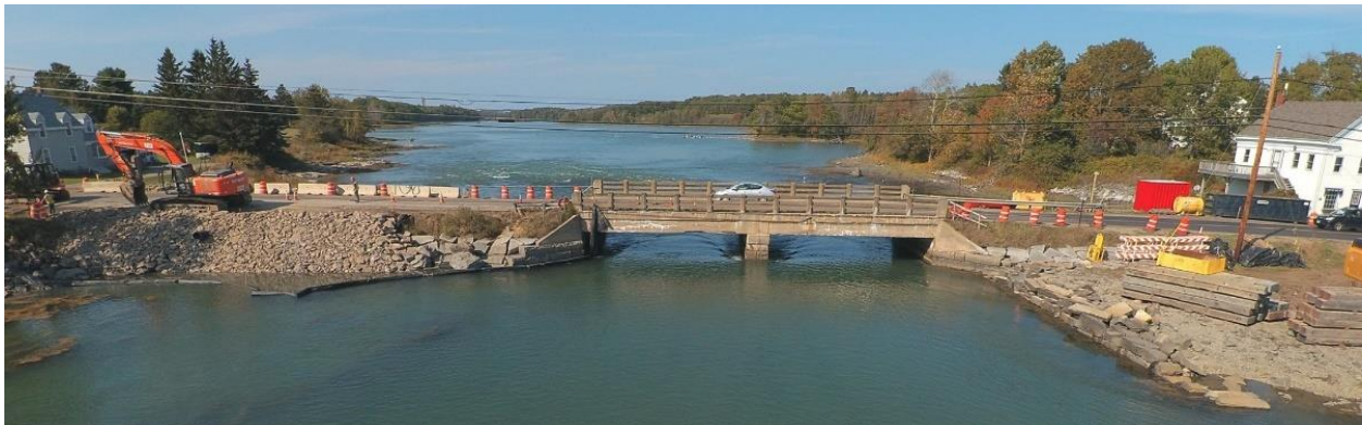
Figure 1 – Site Challenges at the Existing Bridge
