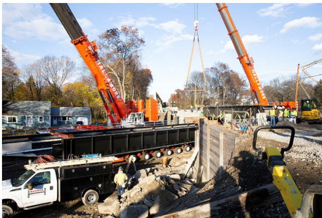
Photo #14: Bridge superstructure erection
