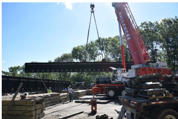
Photo #8: A girder is lifted into place in the MassDOT yard off site
