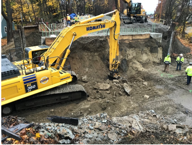
Photo #12: Existing abutment demolition
