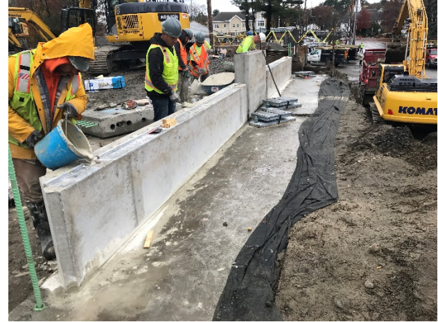
Photo #13: Precast backwall and bearing installation
