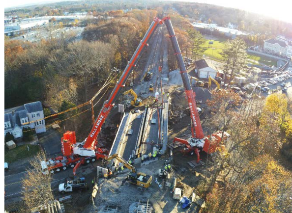
Photo #15: Drone view of superstructure erection
