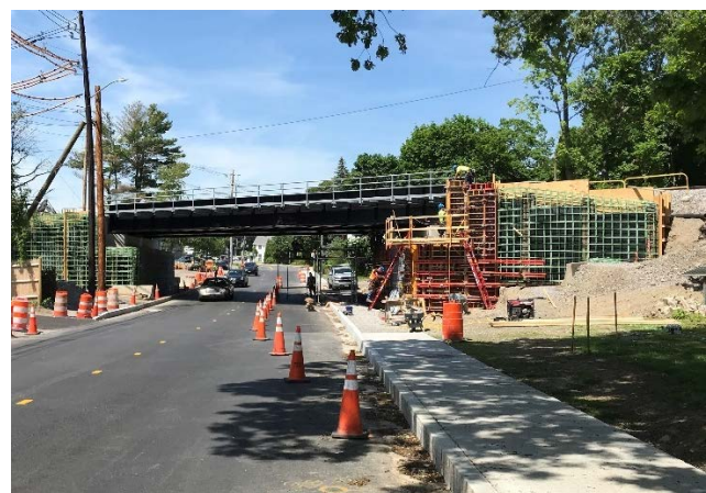
Photo #18: Installation of C.I.P. concrete facing on the soldier pile and lagging walls
