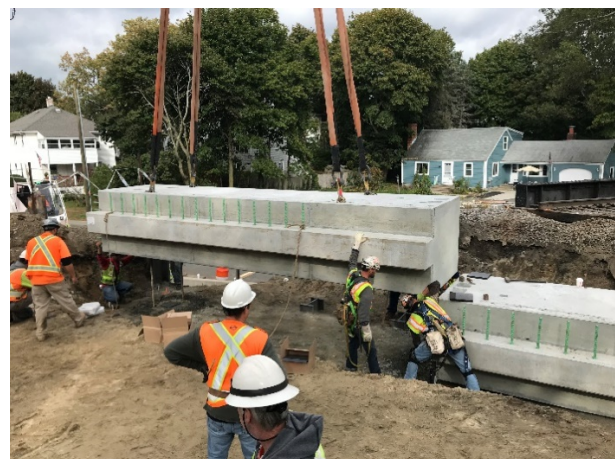
Photo #7: A precast cap is lifted into place on the drilled shaft foundation
