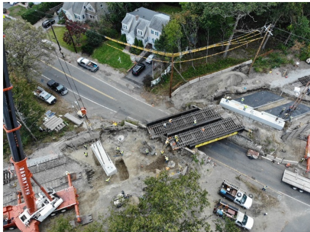
Photo #6: Drone view of substructure installation
