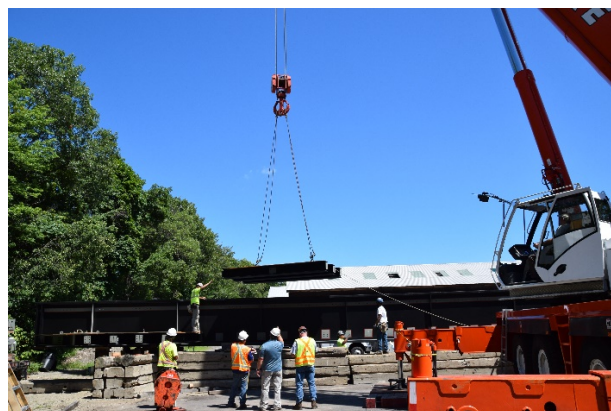
Photo #9: A floorbeam and deck plate section is lifted into place with the braced girder
