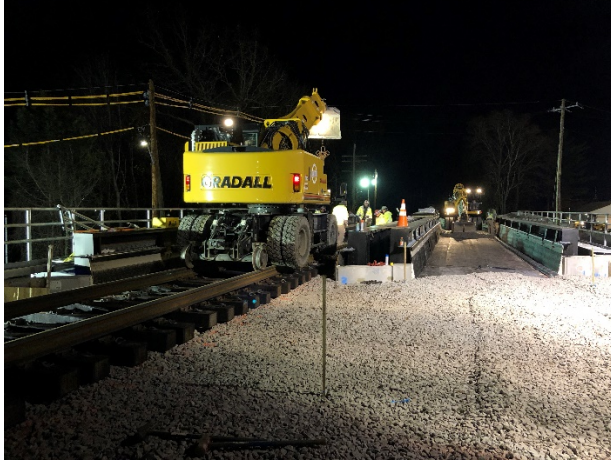
Photo #15: Final track work on bridge
