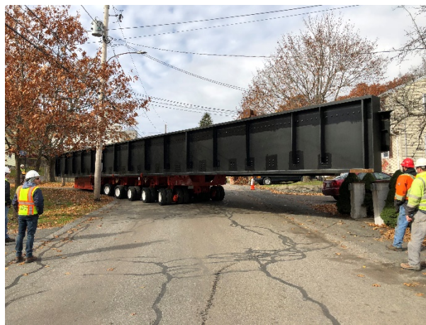
Photo #11: The SPMTs maneuver around a tight corner on the way to the bridge site
