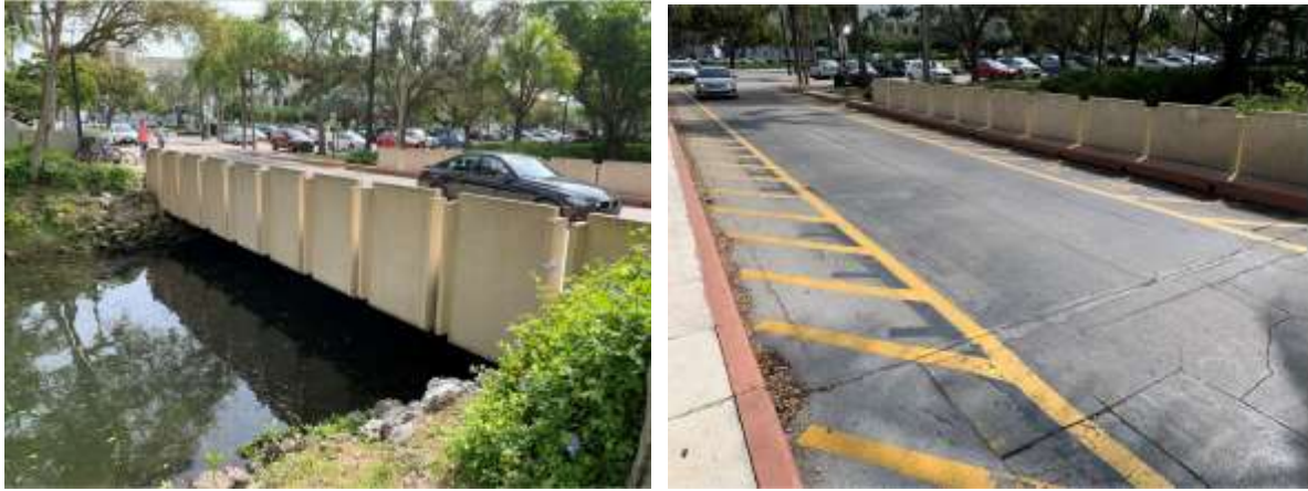
Figure 5: College Drive Bridge, University of Miami
