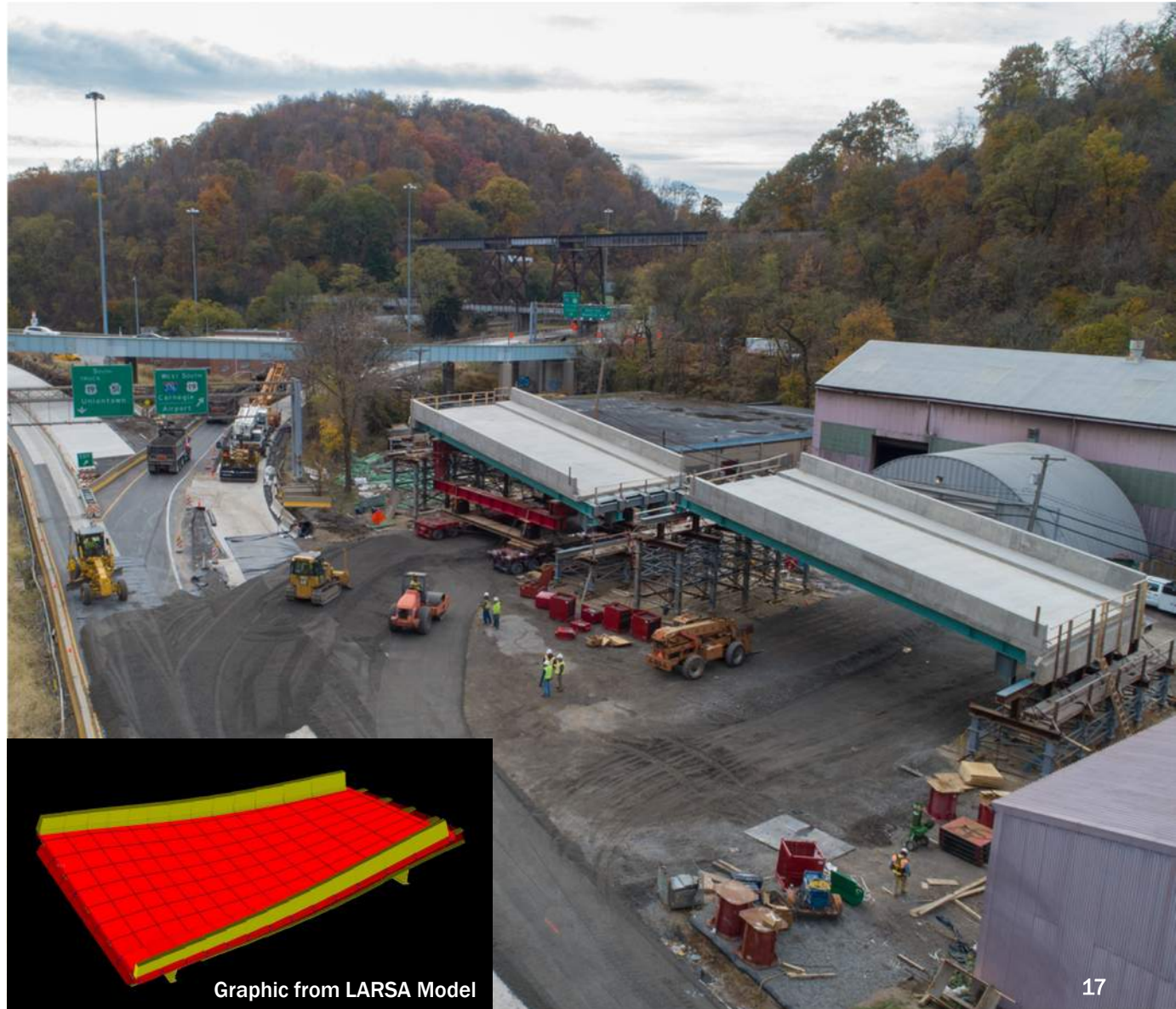
PennDOT's First SPMT Bridge Move: Shaler Street Bridge
