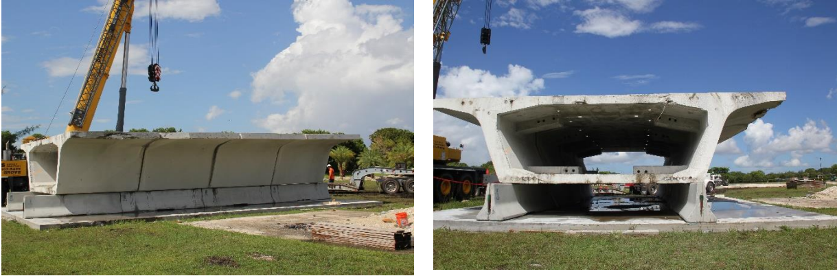
Figure 1: Segments of segmental concrete bridge at FIU.
