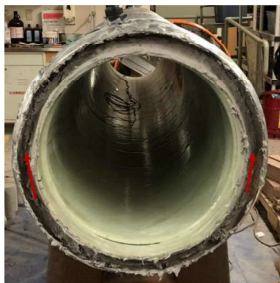
Figure 3. GFRP Slipliner using wood spacers [3]
