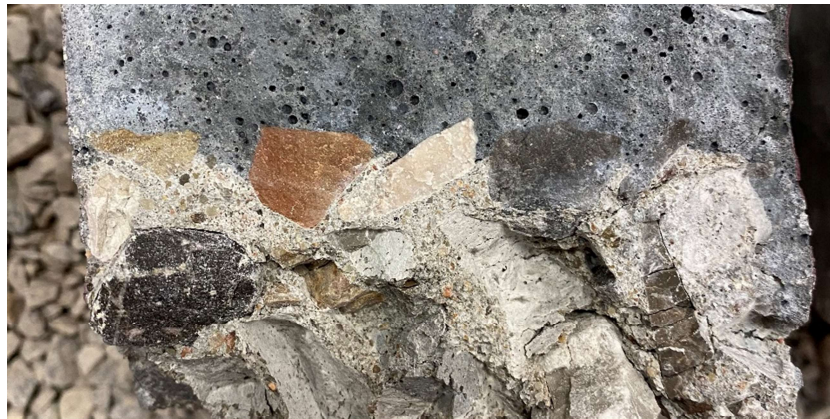
Figure 25. UHPC-conventional concrete interface for failed specimen shown in Figure 24
