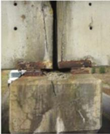
Corrosion of substructure under expansion joint
