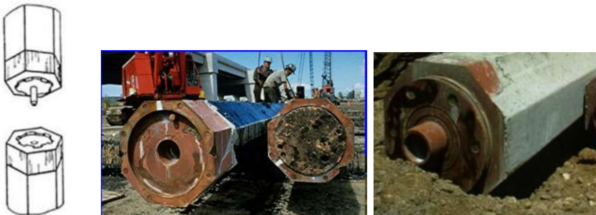
Figure 20: Mechanical splice (Mullins & Sen, 2015)
