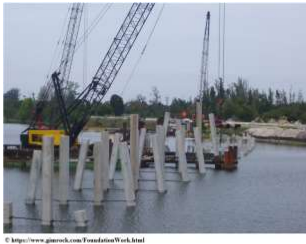
Figure 7: Prestressed-Precast Concrete Piles in marine environment
