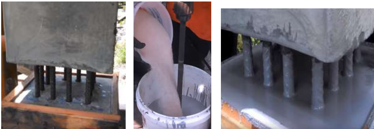
A: Step 1: Inserting dowel rebars B: step 2: Filler or bonding material C: Step 3: Final installation
