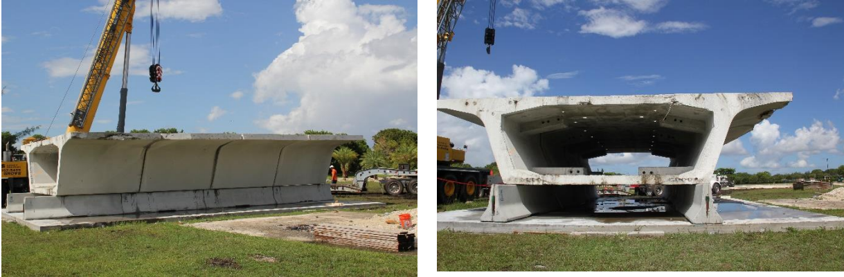
Figure 1: Segments of segmental concrete bridge at FIU.
