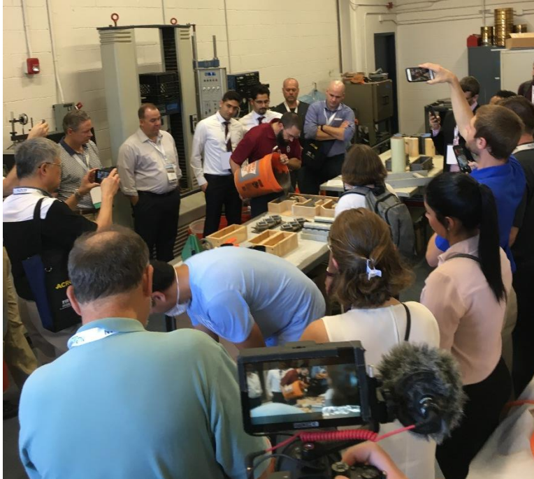
Figure 26. Placement of non-proprietary UHPC in demonstration formwork during the mixing and placement demonstration workshop at FIU
