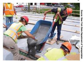
Figure 4. UHPC being placed into an expansion joint (NYSDOT)
