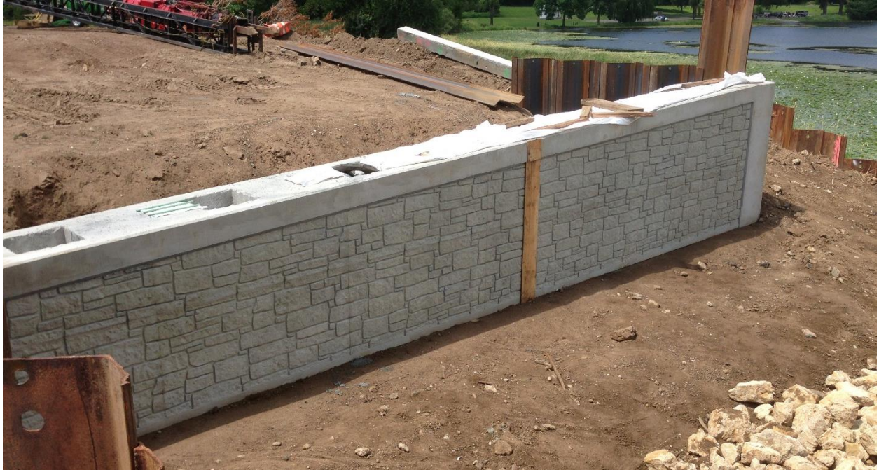
Figure 11. Precast abutment set showing pile grout pockets with wingwalls that consisted of a permanent sheetpile wall with a CIP facing and top coping
