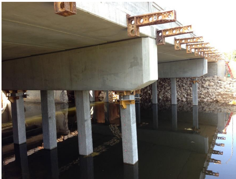
Figure 9. Keller Lake precast concrete bridge construction including inverted-T geometry (top)
