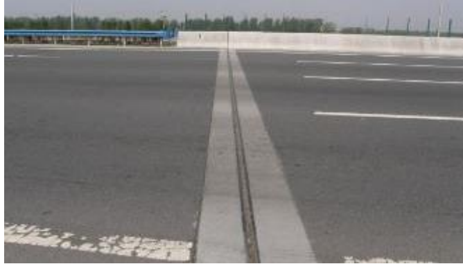
Figure 2.4. Typical strip seal joint
