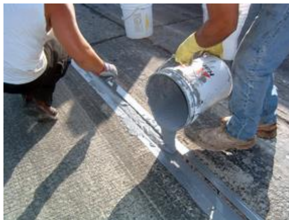
Figure 2.17. Elastomeric concrete for expansion joint repair
