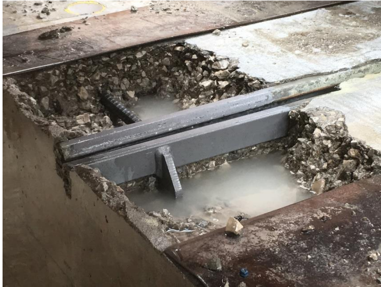
Figure 5.16. Hydrodemolition progress
