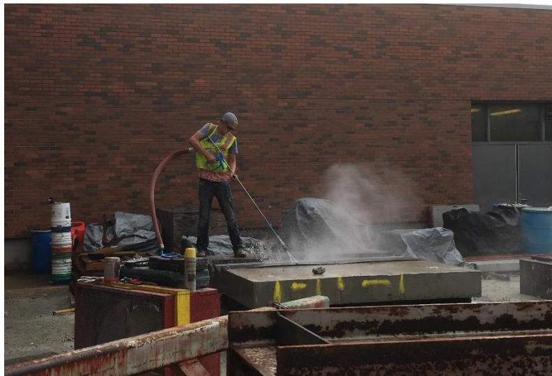
Figure 5.17. Cleaning the joint after hydrodemolition
