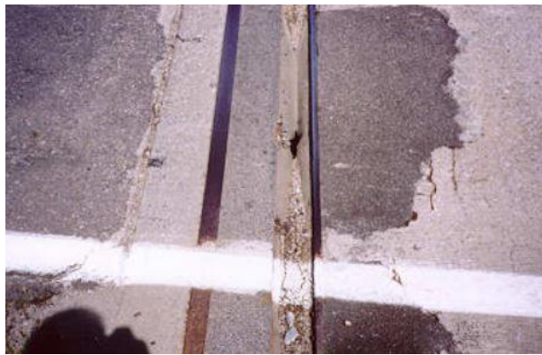
Figure 2.5. Strip seal joint with punctured gland
