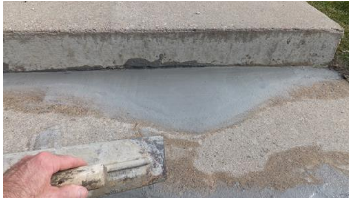
Figure 2.16. Magnesium phosphate cement being used for patching
