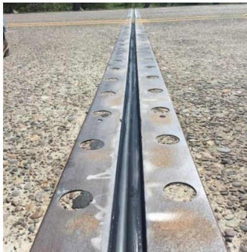
Figure 2.7. EMSEAL BEJS retrofit installed
