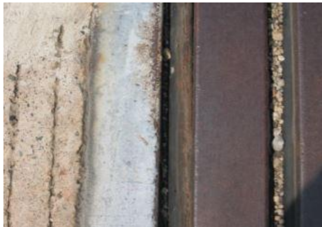
Figure 2.12. Modular joint with debris, preventing closure
