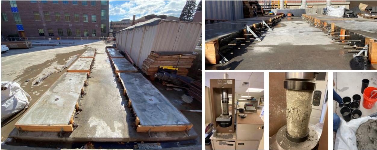
Figure 19 – Deck panels' construction, reinforcement, and cast concrete
