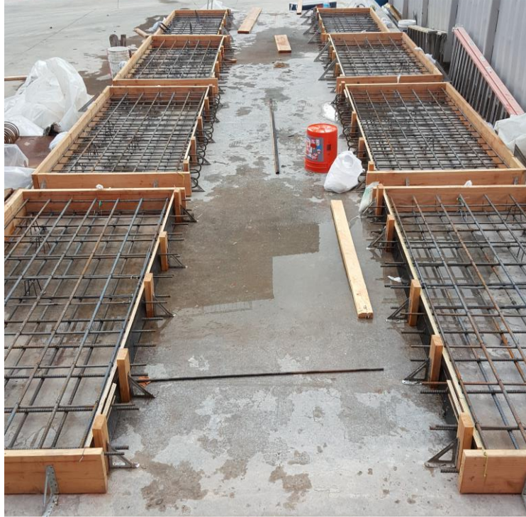
Figure 18 – Formwork and reinforcement for construction of deck panels and specimens
