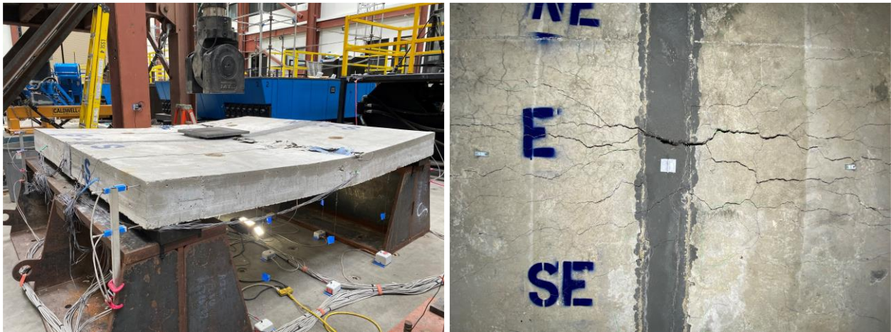
Figure 24 – Damage scheme of specimen S2.
