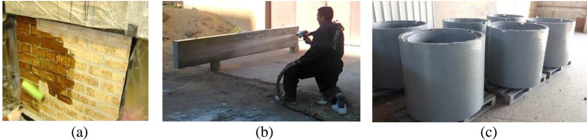
Figure 1: Application of polyurea coating (a) masonry slab (photo is taken from [6]), (b) RC beam specimens (photo is taken from [12]), and (c) concrete pipe (photo is taken from [2]).
